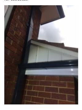
These two photos show the narrow castern eave to the garage, which will need to be tested for asbestos.
