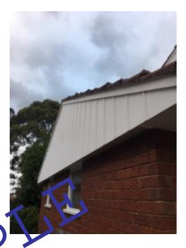
This photos shows the ray in front on the garage, which is sheet material and needs to be tested for asbestos.
