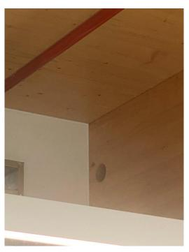
50. In various locations, the painter has poorly prepared, painted and cut in on the wall and timber junctions. The painter should remove all excess mastic, sand and prepare the plasterboard and create sharp, crisp lines within the paintwork.
