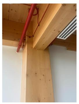
42. There are splits within the timber cladding applied to the undersie fo the dropdoiwn beams.
