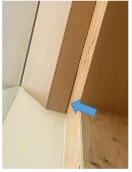
The ceiling and column junction has excess gaps due to poorly cut and installed timber
