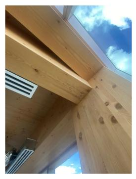
35. Clear coat runs can be seen to be dripping off the underside of the dropdown beams, seen within the image below. A light rub down to remove the lacquer that has bubbled, possibly due to excess lacquer being applied in the one application.
