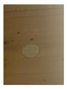
33. The timber beams have been plugged with the incorrect timber, as seen within the image below. There are approx. six locations which need new timber plugs installed.
