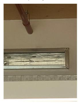
47. Ceiling panels have been installed with butt joints and no glue nor fixings are seen within the joints, however, there are areas within the roof which show excess glue coming through the timber joints.
