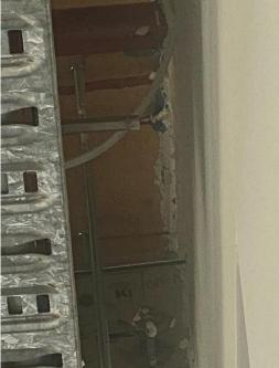
52. Above the shopfront / office front, the wall and timber beam junctions showcase excess mastic between the wall and underside fo the beam, and it also shows poor painting skills as the lines are not straught nor crisp as epxected within a new build.
