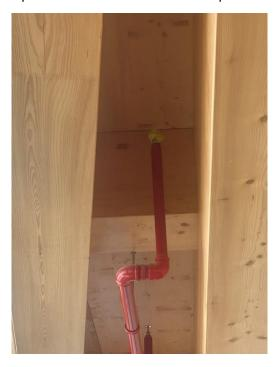
37. Poorly patched and selected materials used to the underside of the ceiling beams, as highlighted within the two images below.
