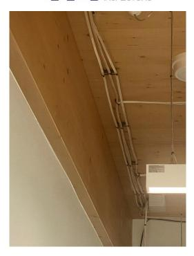
47. The dropdown beams have had holes drilled through them which have compromised the structural integrity of the beams and they have not been plugged matching the remaining holes that were plugged within the other beams.
