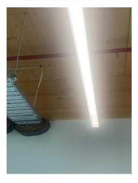
31. There is, randomly found throughout the entire property, paint splash marks on the electrical cables, as seen within the image below, there is a white smear of paint and / or plaster on the red cable on the ceiling elevation.
