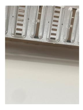
40. Along the wall dividing the office suite and the hallway, the painter has poorly cut in the paintwork which has smeared on the timber ceiling linings.
