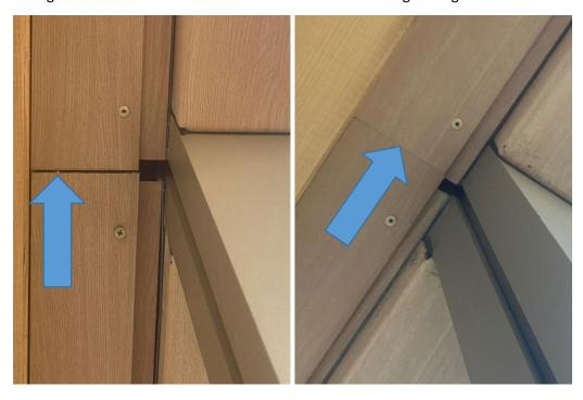
25. Within the images below, it highlights inconsistent gaps and quirks throughout the ceiling panels. Some have a gap of 2mm, and some have a gap up to 5mm. New ceiling panels are required in order to achieve a consistent and professional finish, as currently the gaps range from 0mm, 2mm, 3mm and 6mm.
