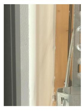
43. Timber dropdown beams have been plugged with the incorrect timber, white plugs were installed within the yellow timber, new plugs with matching timber colour and grain are required.
