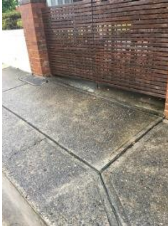
Cracked concrete layback / crossover
