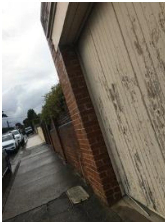
Missing bricks and damaged brick pillar
