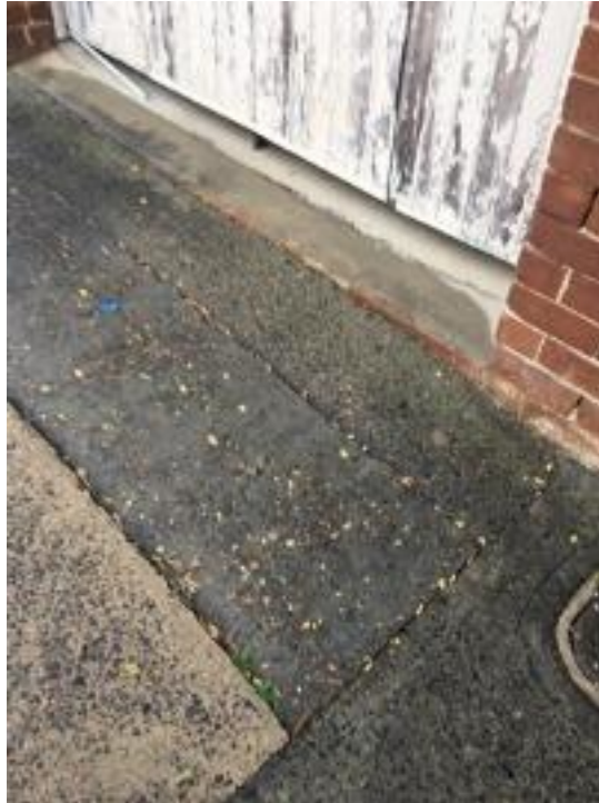
Cracked concrete / footpath
