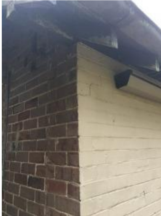
Cracks in the mortar joints within the rear elevation of the house
