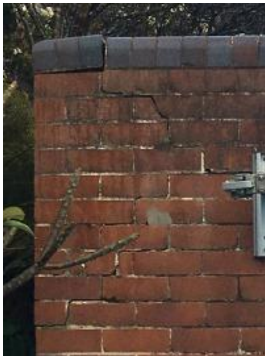
Major structural cracks within the garge structure
