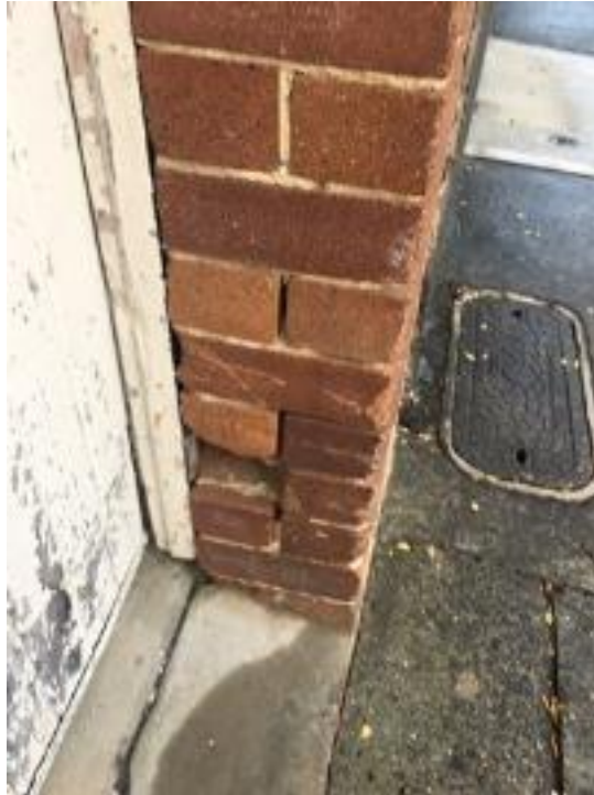
Missing bricks and damaged brick pillar
