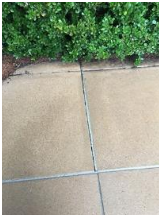
Cracked grout within the pool concourse tiles
