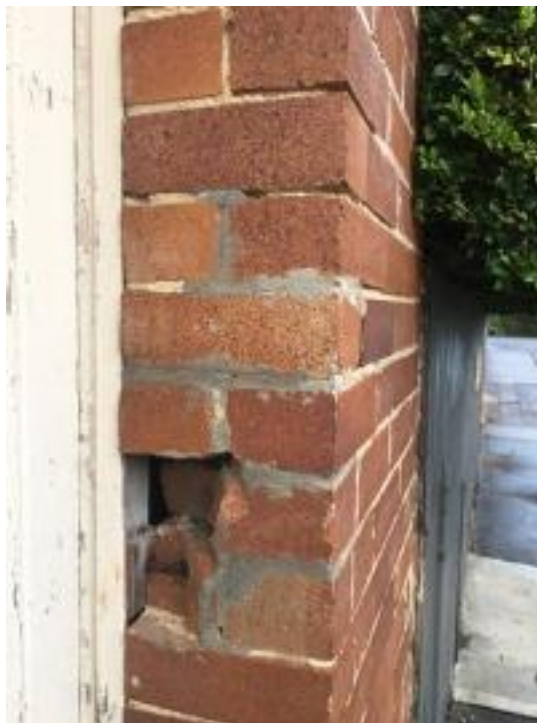
Missing bricks and damaged brick pillar
