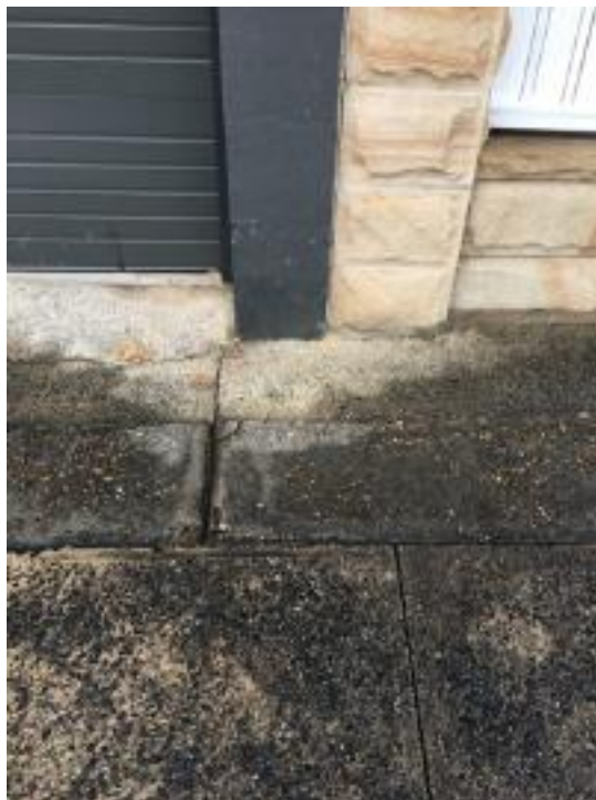
Cracks in the concrete layback and footpath
