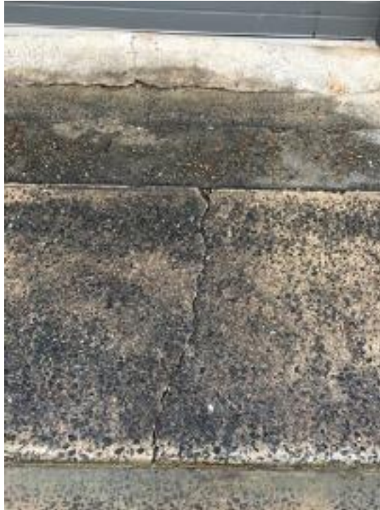
Cracks in the concrete layback and footpath
