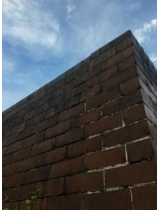
Existing cracks within the brick mortar joints within the street elevation of the garage structure
