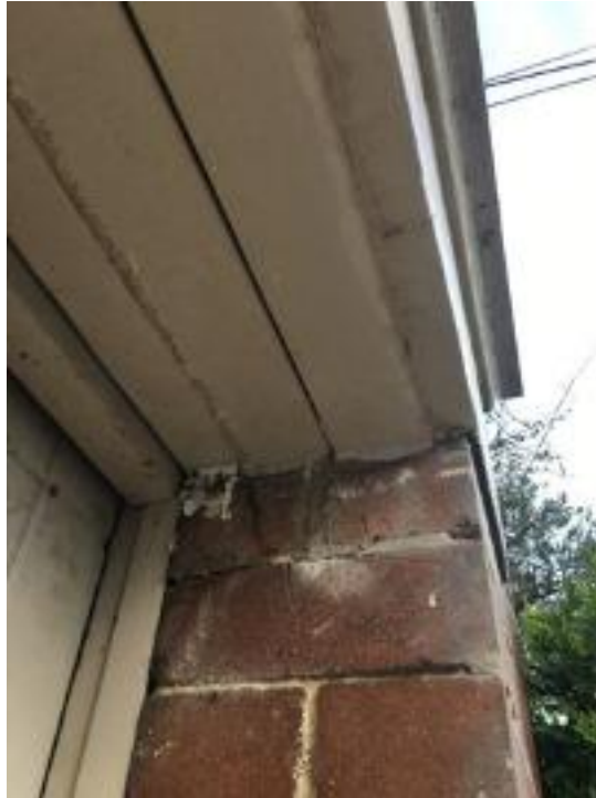
Cracked bricks within the street elevation garage pillar
