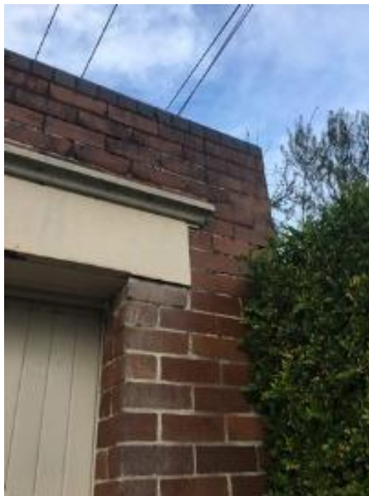
Existing cracks within the brick mortar joints within the street elevation of the garage structure
