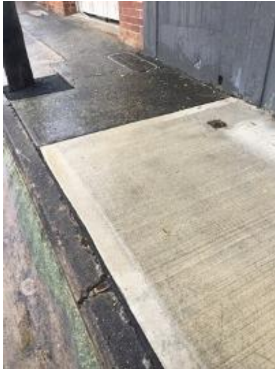
The curb and gutter are defective / cracked
