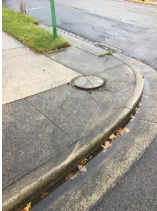
Existing footpath condition in the junction of Fairfax Road and Tivoli Street Mosman (Minor cracks)
