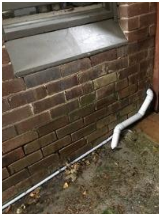
Cracks in the window sills / render, and missing mortar within the face brickwork
