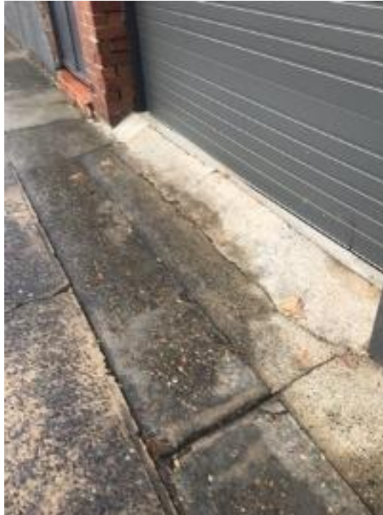
Footpath has excessive cracks within the old and new concrete footpaths
