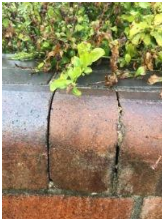
Existing cracks within the brick mortar joints of the brick pillars
