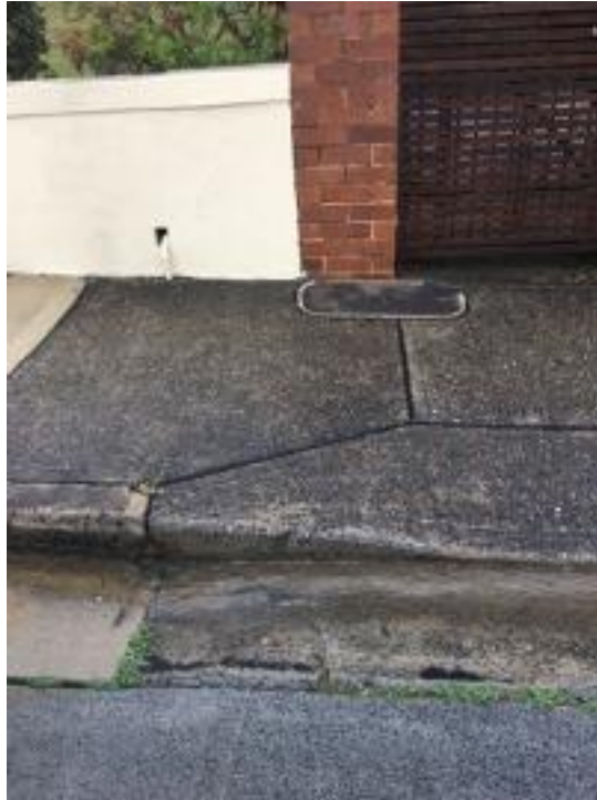
Cracked concrete apron and layback / driveway
