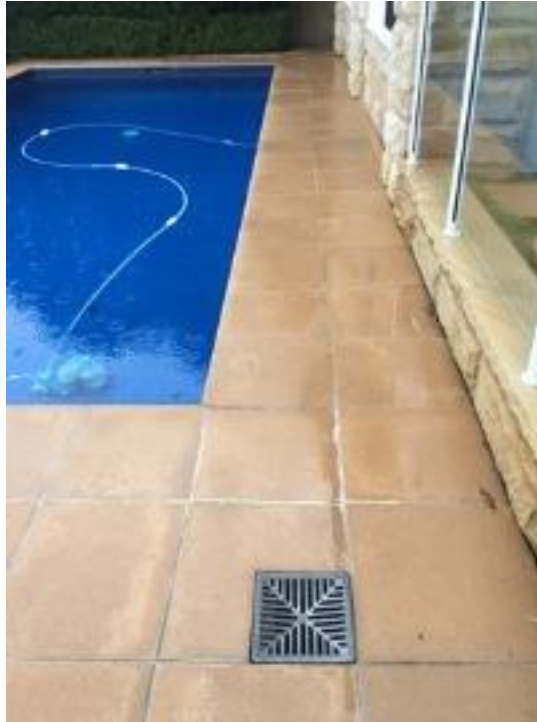
Efflorescence leaching out of the floor tiles and mortar joints within the pool concourse
