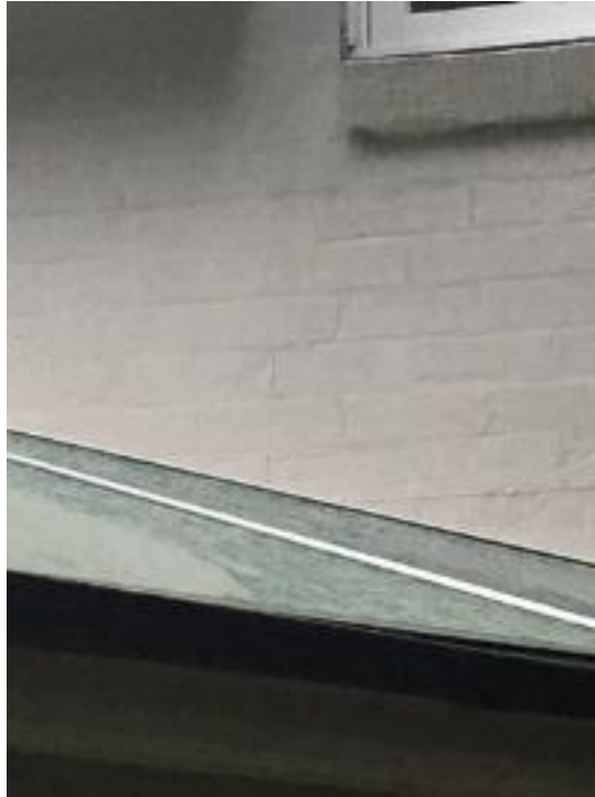
Minor cracks in the rear elevation masonry walls above the roof line
