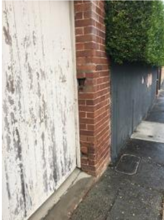
Missing bricks and damaged brick pillar
