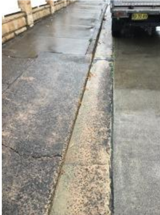
Cracks in the concrete curb, gutter and footpath
