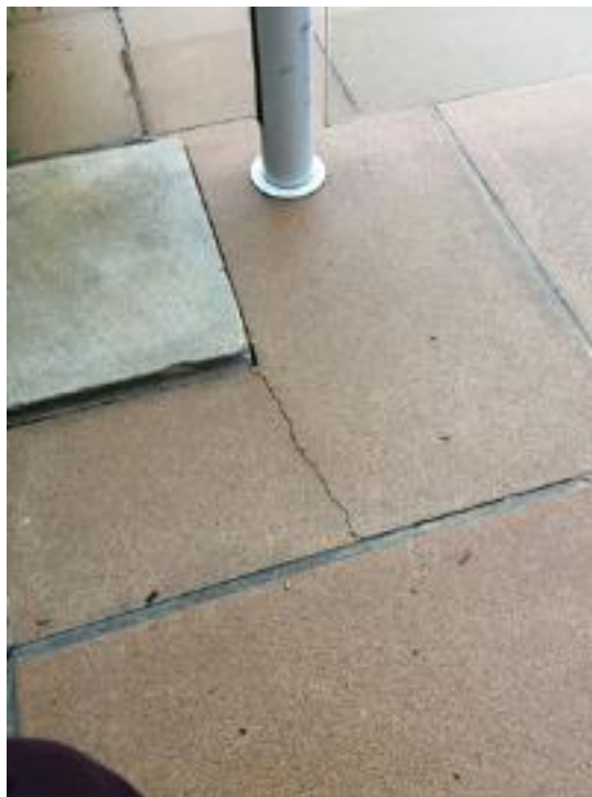
Minor cracks in the pool coping and pool concourse tiles
