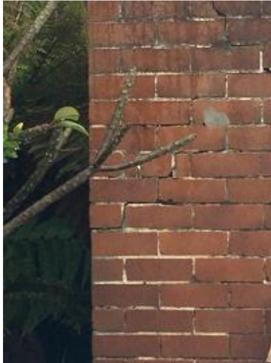
Major structural cracks within the garge structure
