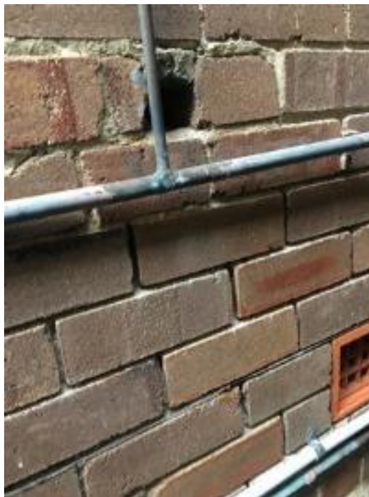
Missing mortar within the face brickwork, right elevation of the house
