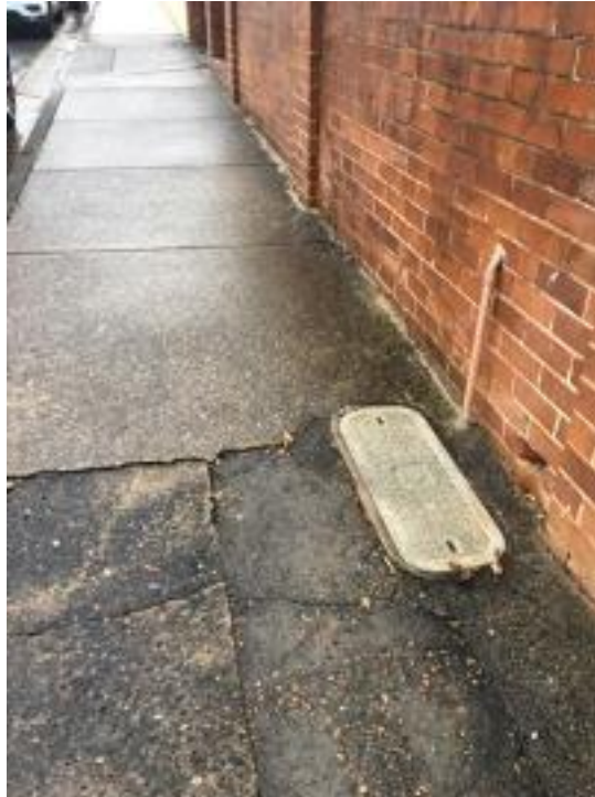
Cracked concrete footpath, driveway and layback
