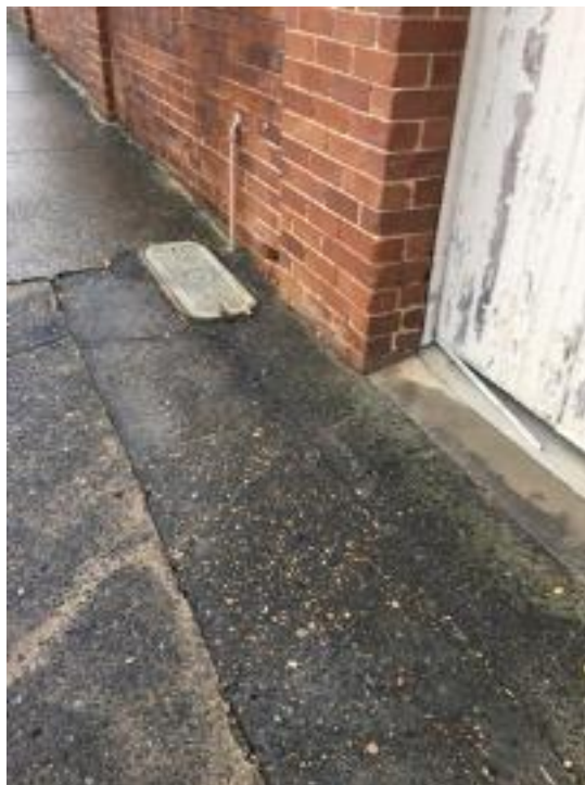
Cracked concrete / footpath
