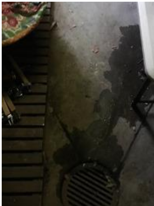
Water ingress within the garage floors, walls and roof structure
