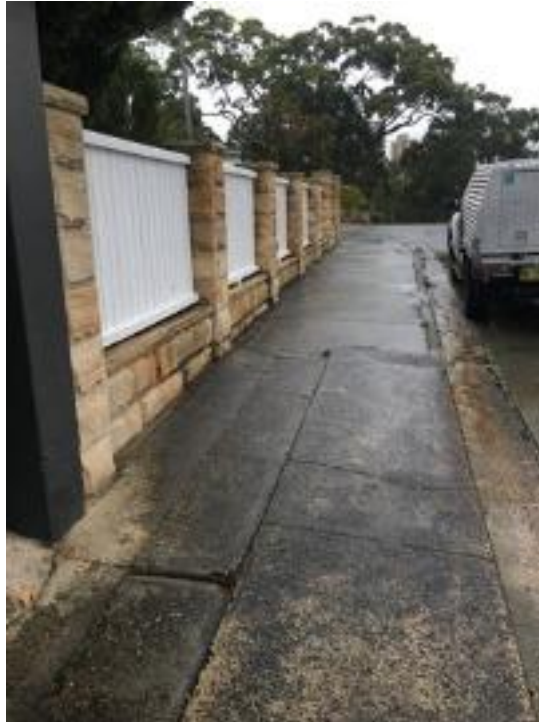
Old / existing cracks / damages in the concrete footpath
