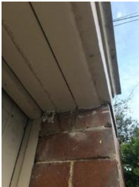
Cracked bricks within the street elevation garage pillar
