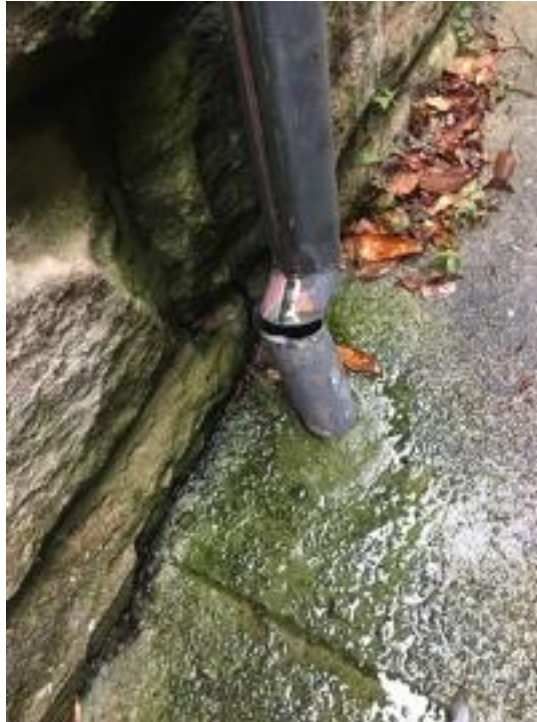
Damaged downpipes
