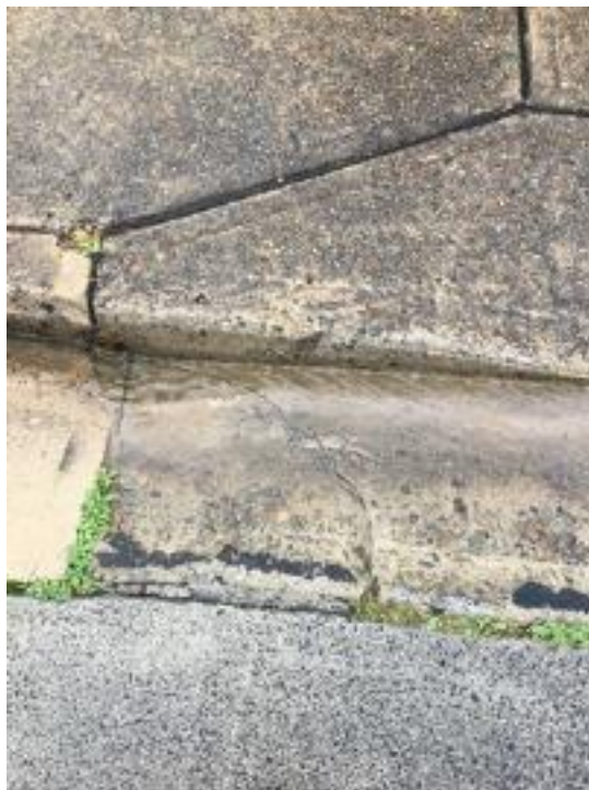
Cracked concrete apron and layback / driveway
