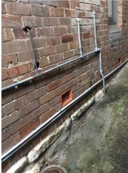
Missing mortar within the face brickwork, right elevation of the house
