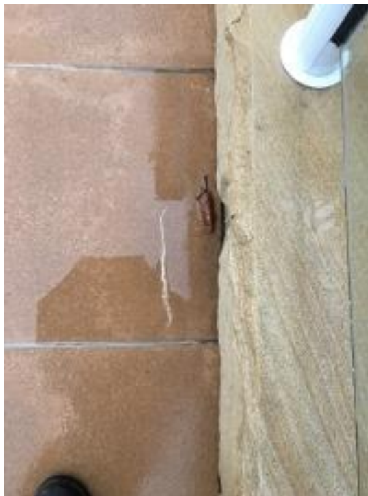
Efflorescence leaching out of the floor tiles and mortar joints within the pool concourse
