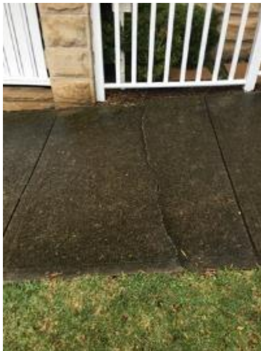
Cracked concrete footpath, out the front door of the property
