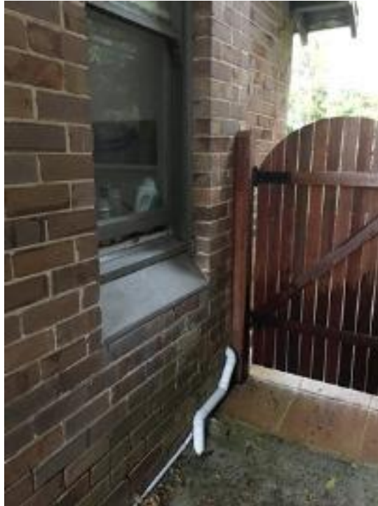
Cracks in the window sills / render, and missing mortar within the face brickwork
