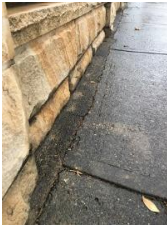
Sunken / subsided concrete footpath
