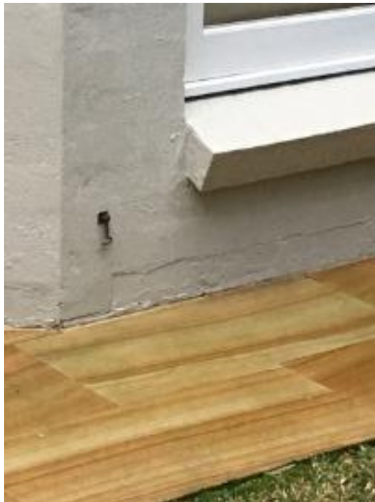
Minor cracks in the base of the external masonry wall
