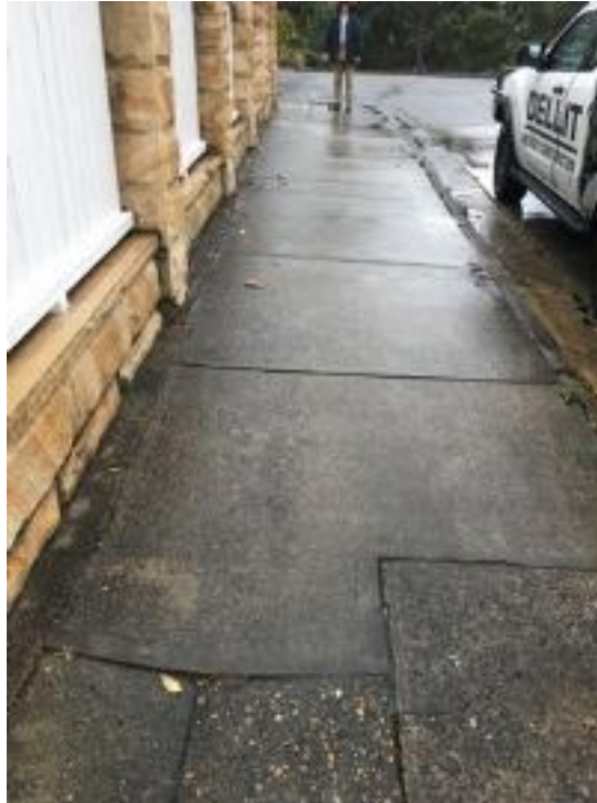
Sunken / subsided concrete footpath
