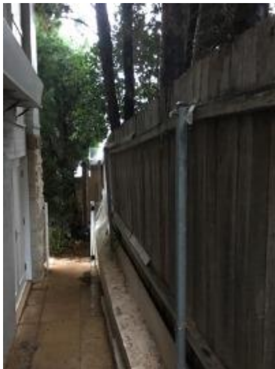
Bowed timber fence and masonry retaining wall
