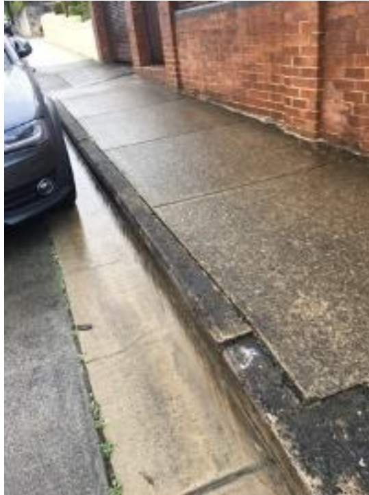
Cracked concrete curb and gutter
