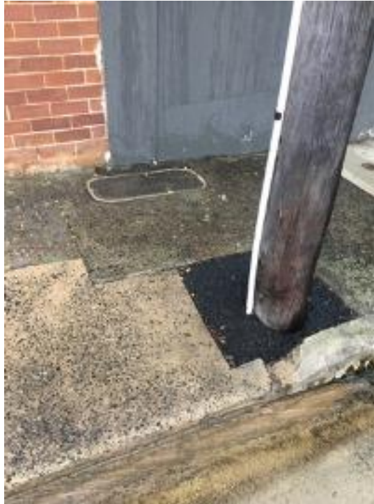
Cracked concrete footpath to the right corner of the footpath, and around the curb and gutter in front of the power pole
