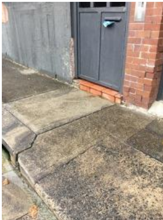
Footpath has excessive cracks within the old and new concrete footpaths
