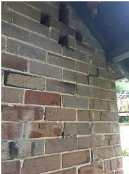
Cracks in the rear elevation / rear right coner of the house
