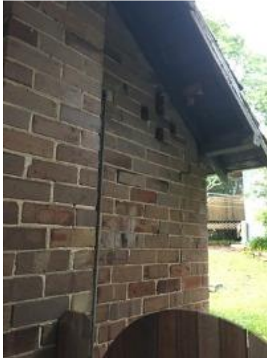
Cracks in the rear elevation / rear right coner of the house
