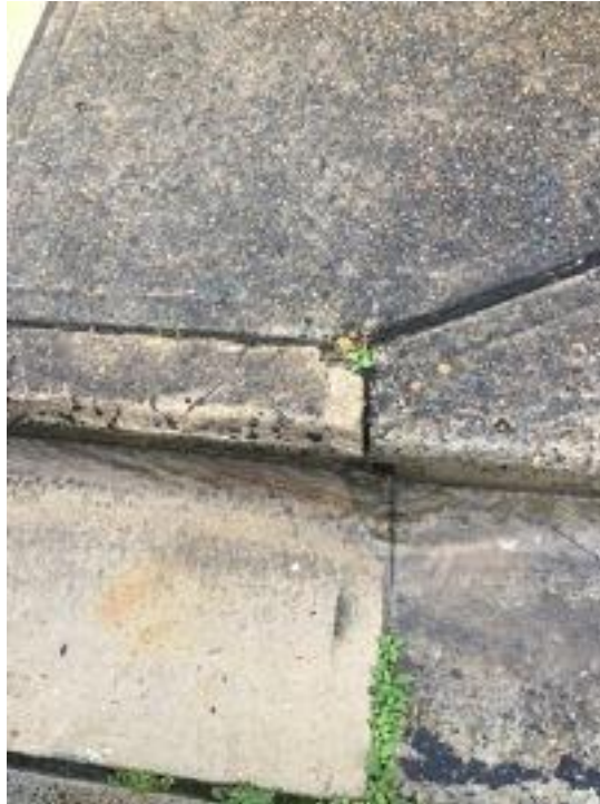
Cracked concrete curb, gutter and layback
