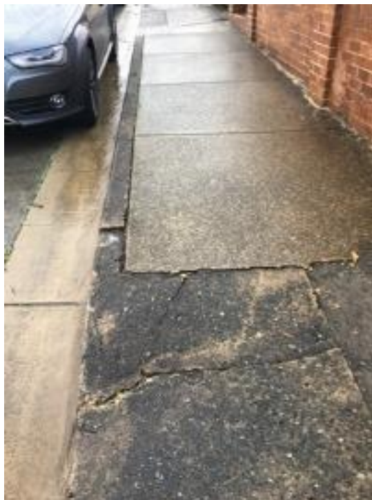
Cracked concrete footpath, driveway and layback
