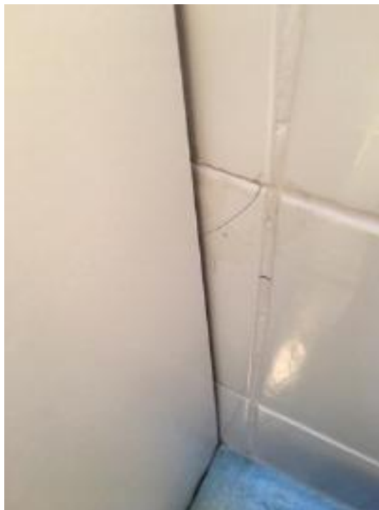
Bathroom wall tiles are chipped and cracked
