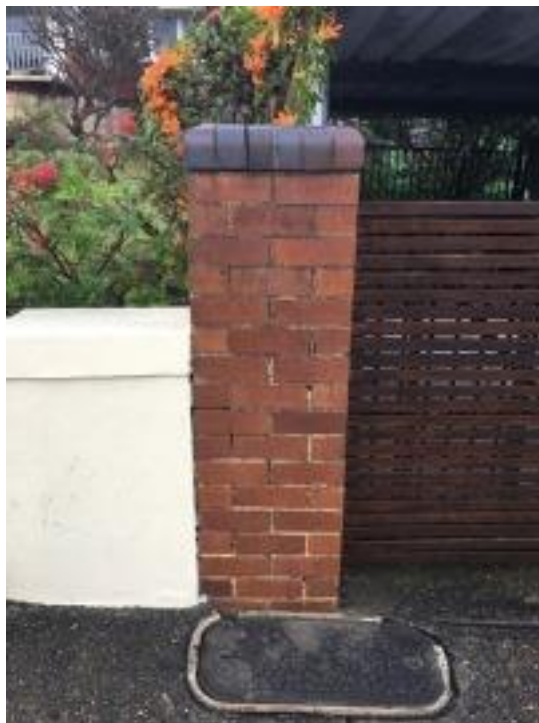
Minor cracks within the face brickwork within the front brick pillar
