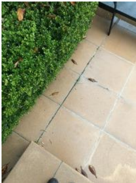
Cracks in the floor tiles and floor tile mortar joints
