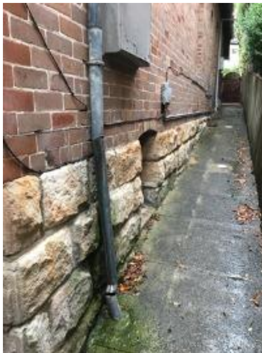
Damaged downpipes
