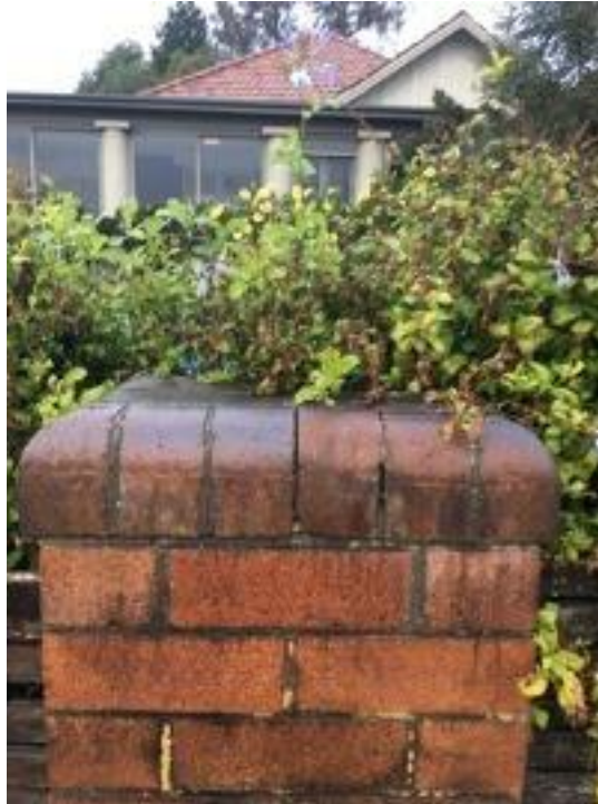
Existing cracks within the brick mortar joints of the brick pillars
