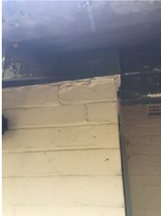
Minor cracks in the brick mortar joints / face brickwork, rear elevation of the house
