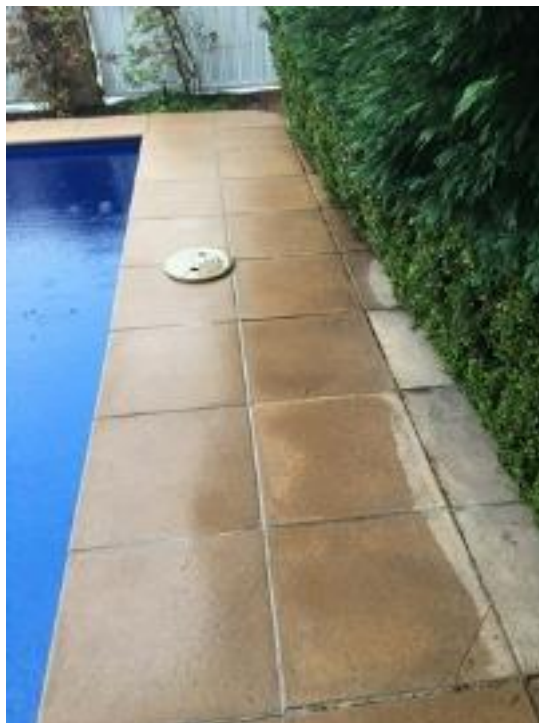
Chipped / cracked pool floor tiles within the pool concourse
