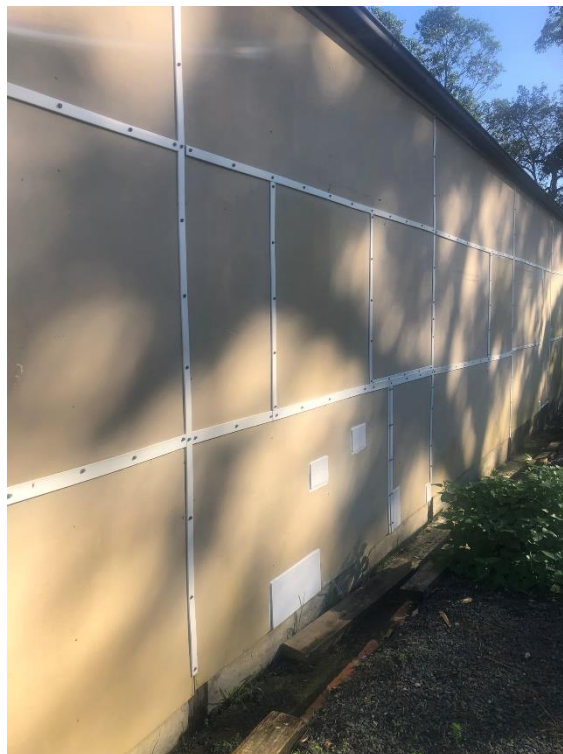
Damaged trimwork and cover panels to the external wall linings.
