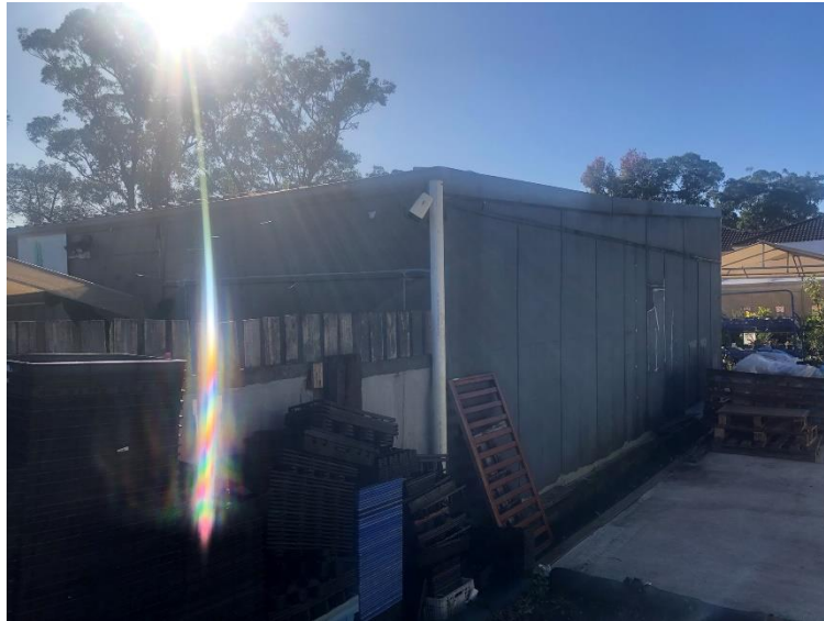
Damaged, cracked and defective fibro and possible asbestos external wall linings. Damaged, cracked and defective gutters and downpipes.
