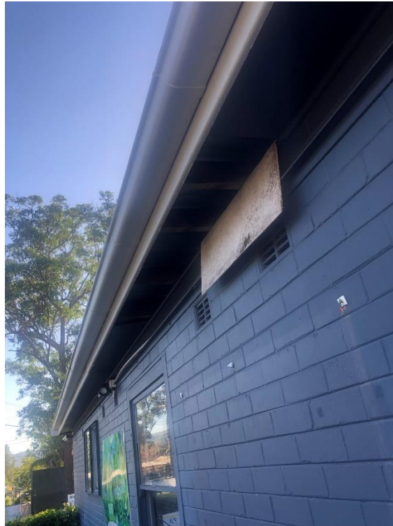
Fallen soffit linings.
