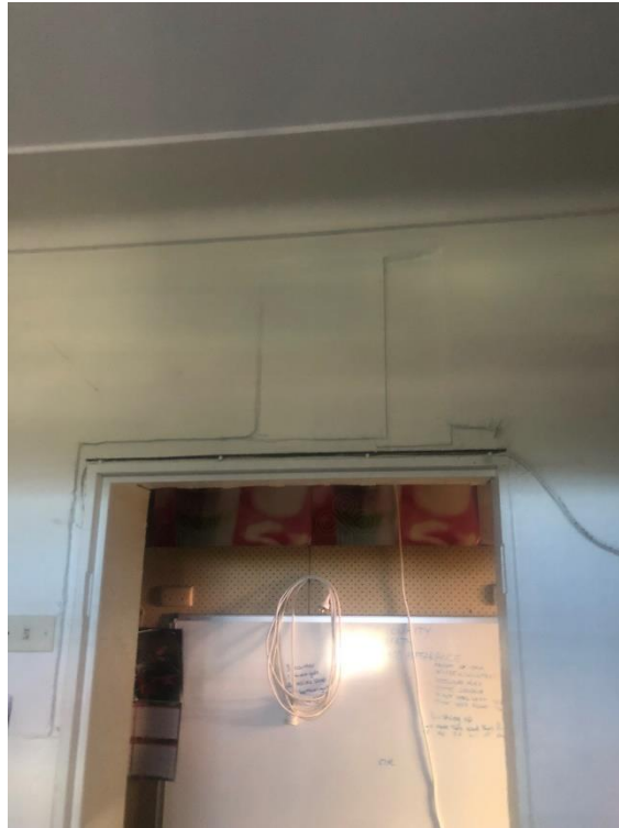
Cracks within the internal wall linings above the door and adjacent to the CCTV camera system.
