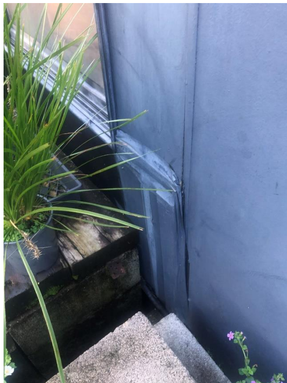
Cracked and damaged fibro / asbestos wall linings.
