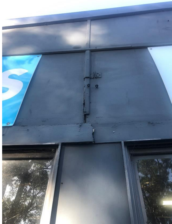
Cracked and damaged fibro / asbestos wall linings above and surrounding the external windows and within the external walls.
