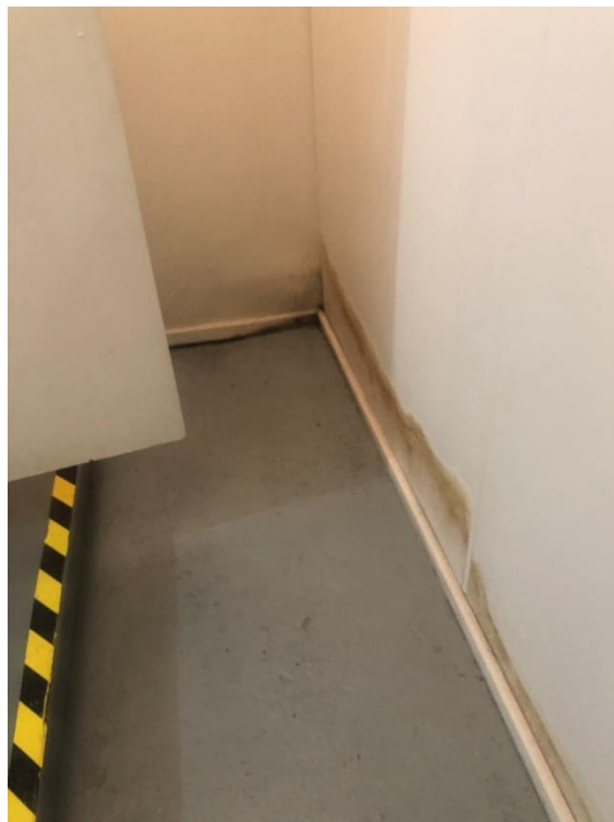
Mould and moisture within the wall linings.
