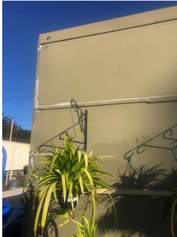
Cracked asbestos / fibro wall linings.
