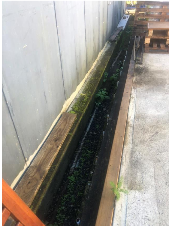
Mould and moisture damage within the concrete slab and external fibro / asbestos wall linings. Cracked and damaged fibro / possible asbestos wall linings.
