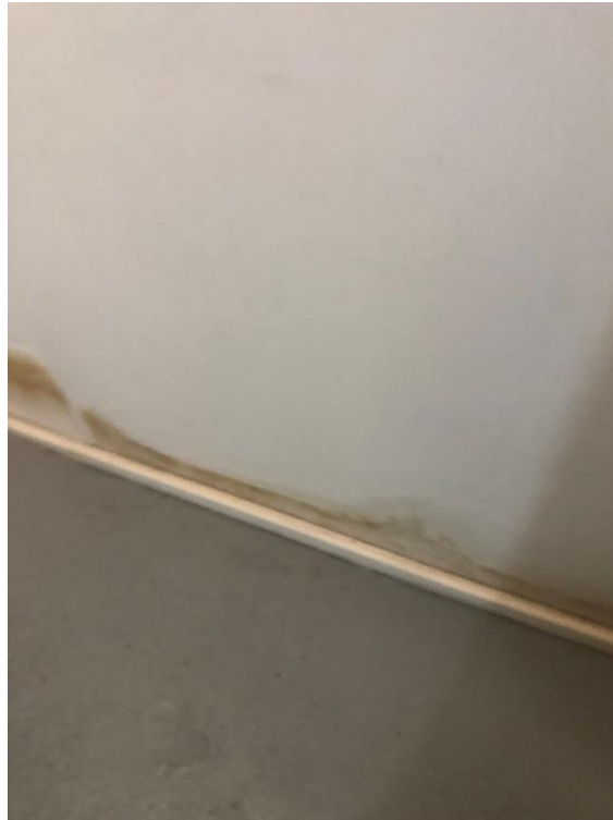
Mould and moisture within the wall linings.
