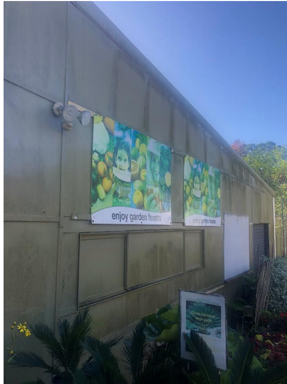
Cracked asbestos / fibro wall linings. Damaged and leaning steel structure with lightweight canopy.
