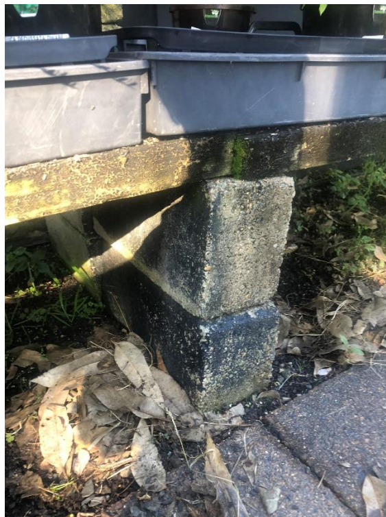
Subsided pavers and elevated shelves, sagging and damaged.
