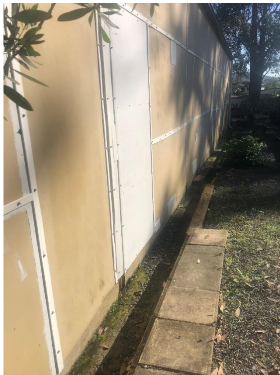
Cracked and damaged wall linings, mould and moisture within the external wall linings.
