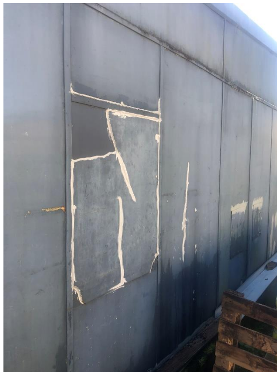
Mould and moisture damage within the concrete slab and external fibro / asbestos wall linings. Cracked and damaged fibro / possible asbestos wall linings.
