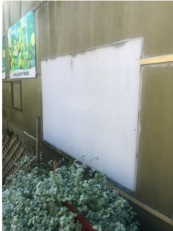
Cracked, damaged and partially repaired fibro / asbestos wall linings.
