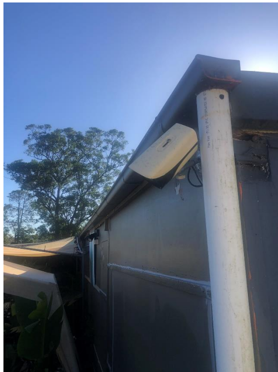
Damaged, cracked and defective fibro and possible asbestos external wall linings. Damaged, cracked and defective gutters and downpipes.
