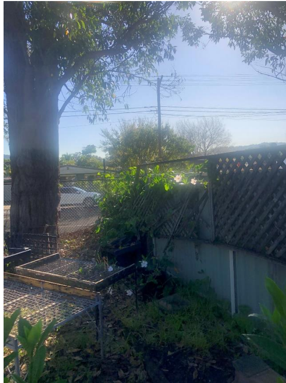
Collapsed lattice, together with damaged fibro wall and fence linings. Subsided pavers and vegetation within the floor pavers.
