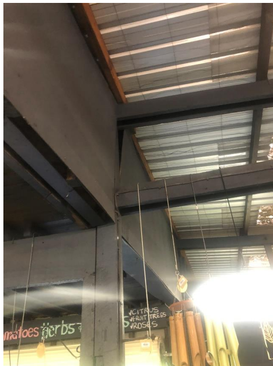
Broken and dmaaged wall linings within the internal elevation of the nursery.
