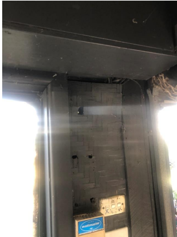
Moisture seen within the internal storeroom walls, ceiling and bulkhead.
