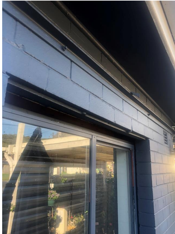
Missing window storm moulds. Damaged wire fencing.
