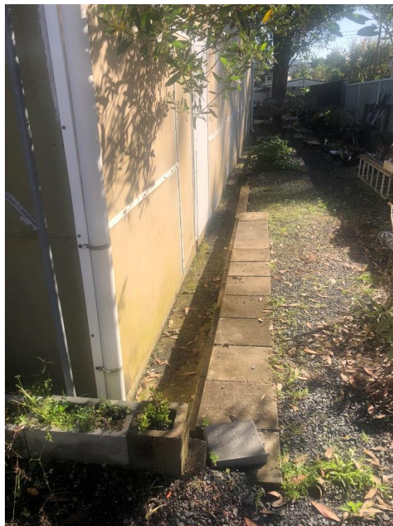
Cracked, damaged and partially repaired fibro / asbestos wall linings.
