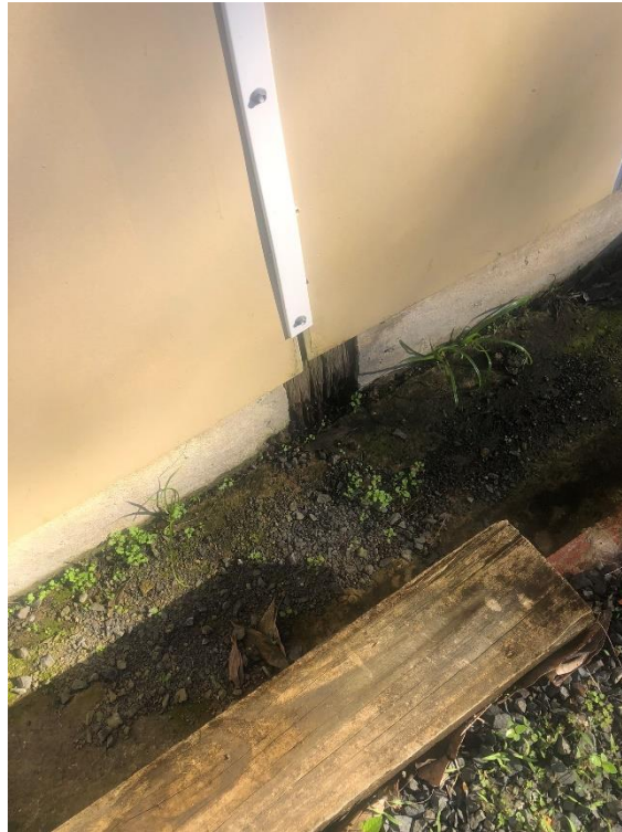
Cracked, damaged and missing fibro / asbestos wall linings and cover panels.
