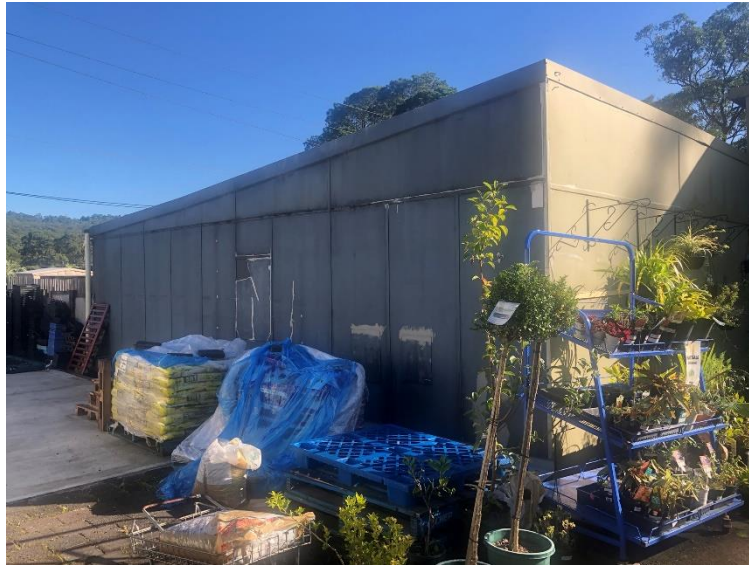
Cracked asbestos / fibro wall linings.
