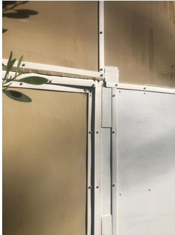
Damaged trimwork and cover panels to the external wall linings.
