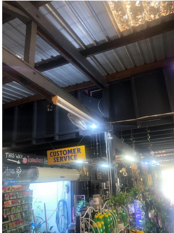
Water entry within the nursery from the roof sheets and skylight junction.
