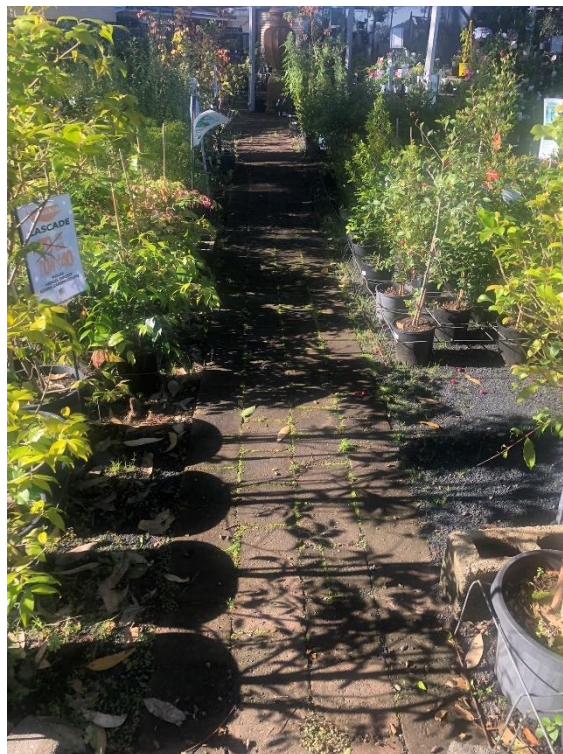
Subsided pavers and vegetation within the floor pavers.
