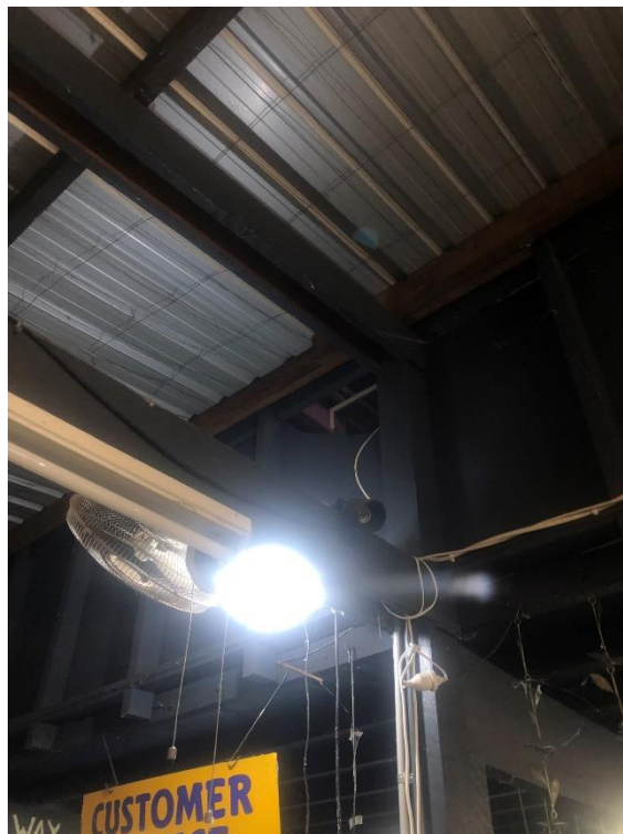
Water entry within the nursery from the roof sheets and skylight junction.
