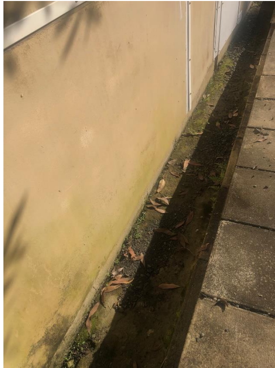
Cracked and damaged wall linings, mould and moisture within the external wall linings.
