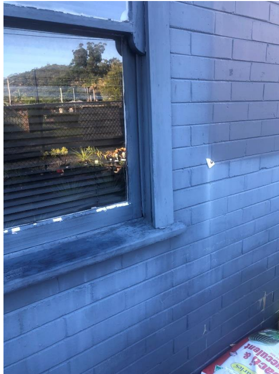
Wood rot within the windowsill, architrave and window unit. Cracked concrete pathways and leaning metal fence line.
