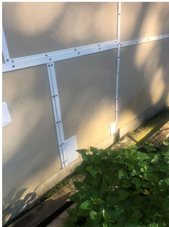
Cracked, damaged and missing fibro / asbestos wall linings and cover panels.
