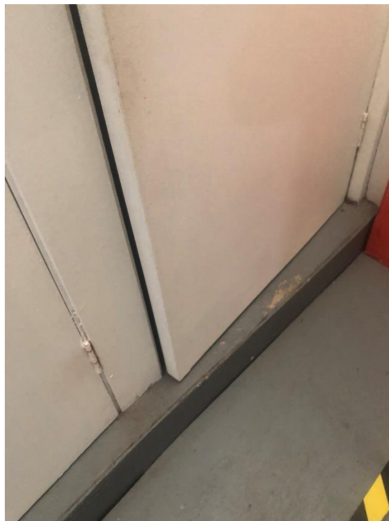
Mould and moisture within the bathroom doors.
