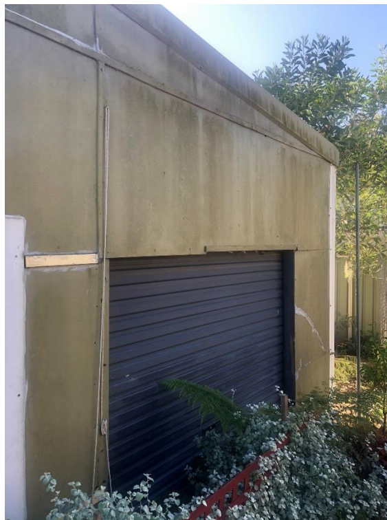
Damaged and leaning steel structure with lightweight canopy. Cracked and damaged fibro / asbestos wall linings.
