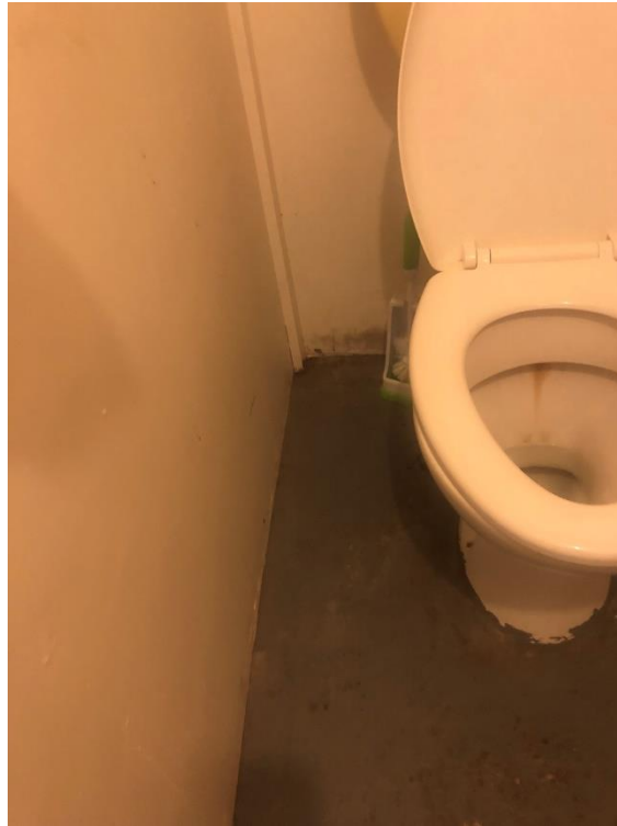
Mould and moisture within the wall linings and floor junctions. Cracks within the bathroom floor.
