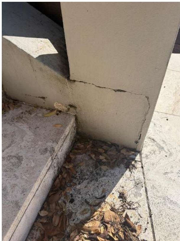
Crack within the staircase side boundary wall and retaining wall junction
