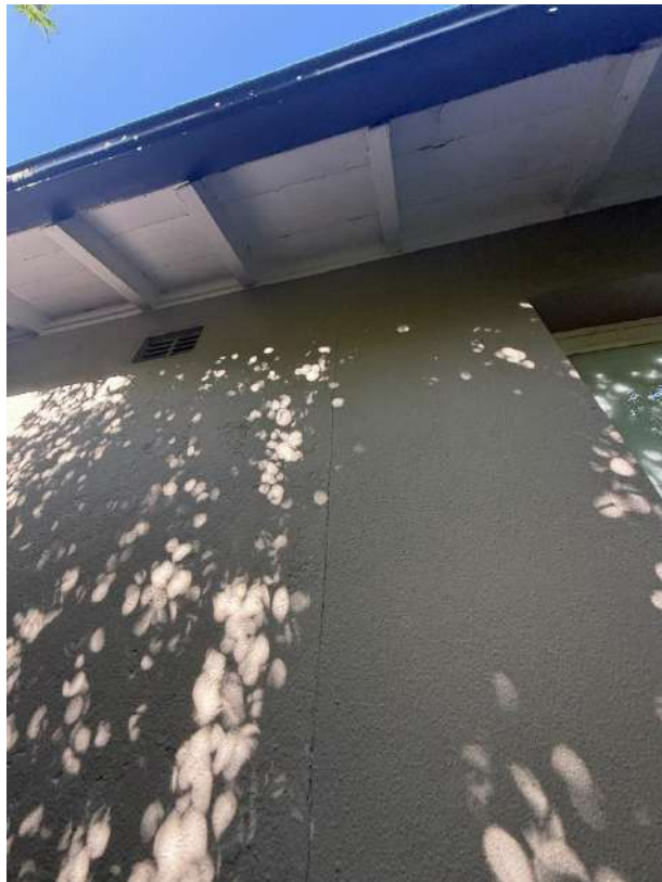
Vertical cracks seen within the external masonry walls running the whole length of the walls from floor to eave linings
