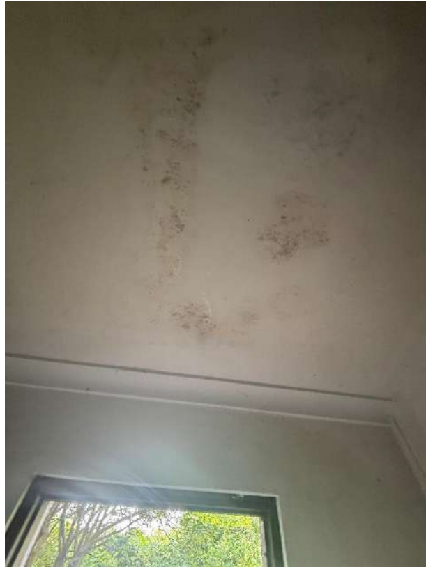
Moisture damage within the ceilings outside bathroom
