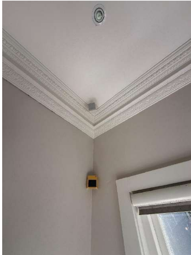
Minor hairline cracks seen within the cornices within the living room ceiling
