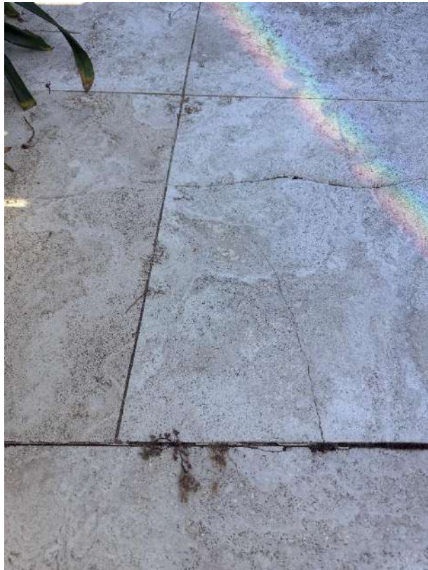
Landing in stairs have cracks through the stone floor tiles
