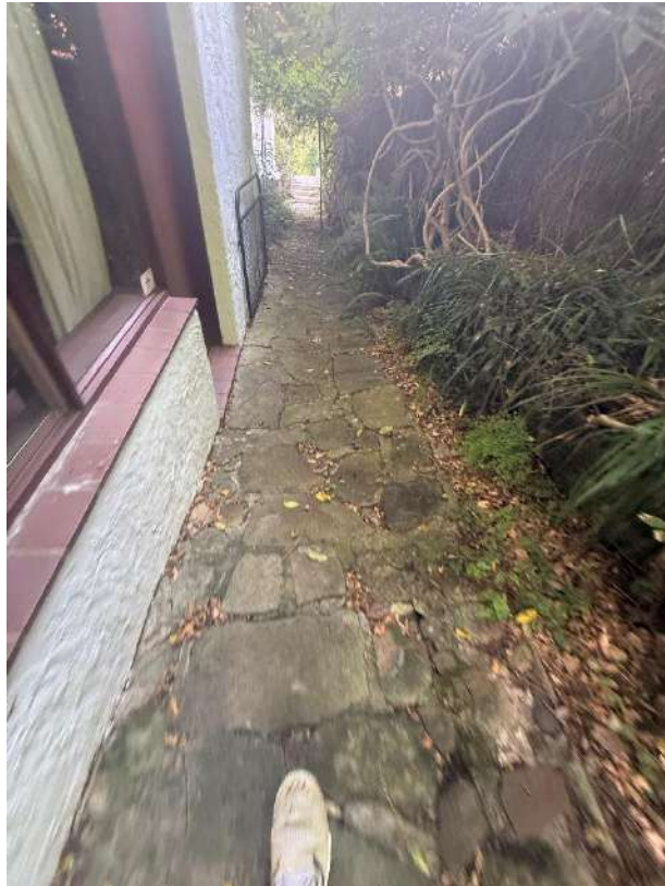
Cracks within the sandstone mortar joints
