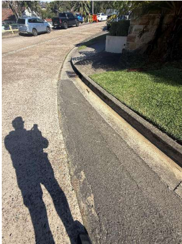
Bitumen cracked
