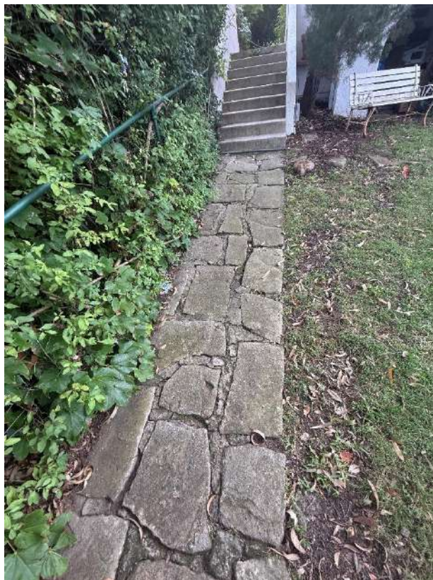
Minor hairline cracks in sandstone flagging floor finish
