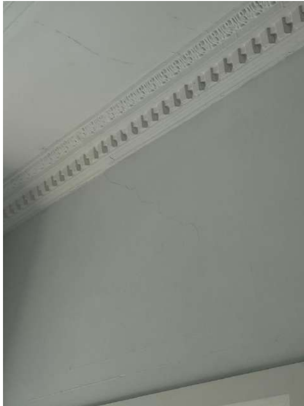
Splayed cracking within the living room walls
