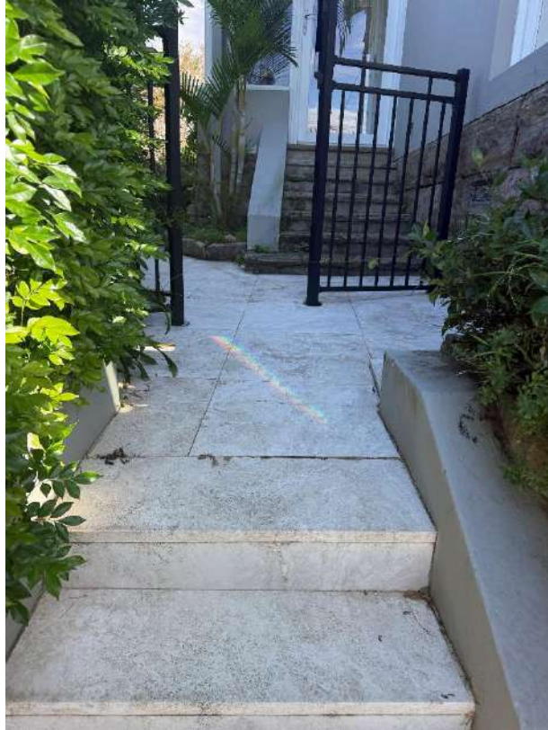
Landing in stairs have cracks through the stone floor tiles
