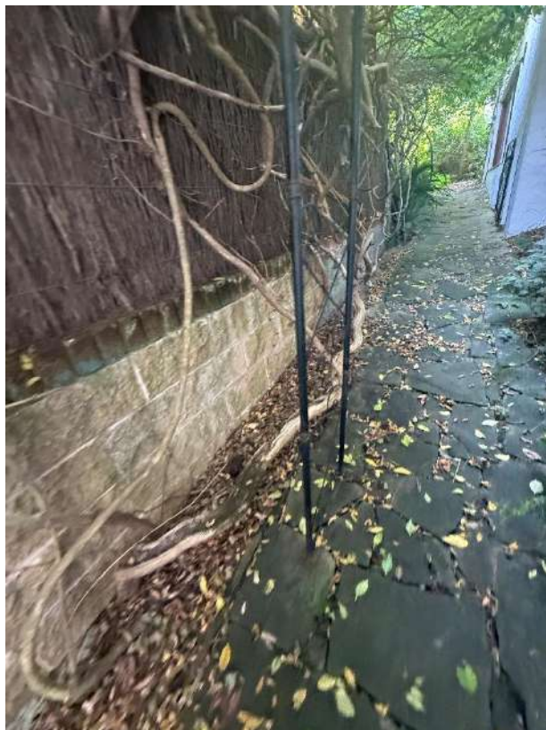
Cracks within the sandstones flagging floor finish
