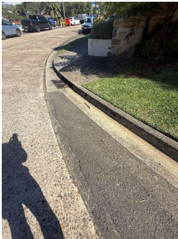
Bitumen cracked
