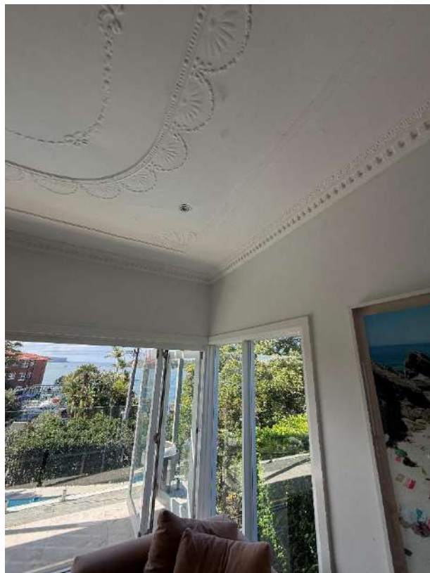
Peeling paint within the living room ceiling and cornices
