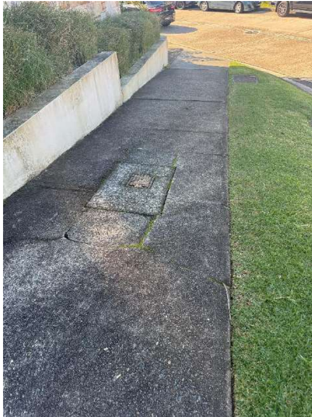
Cracks in the concrete foot path
