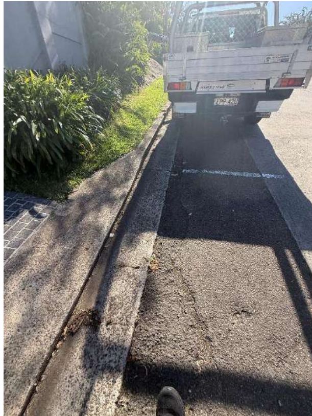
Cracks in curb and gutter
