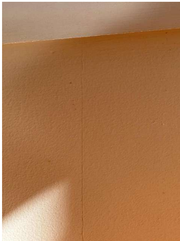
Horizontal cracking within the back office beneath the window frame
