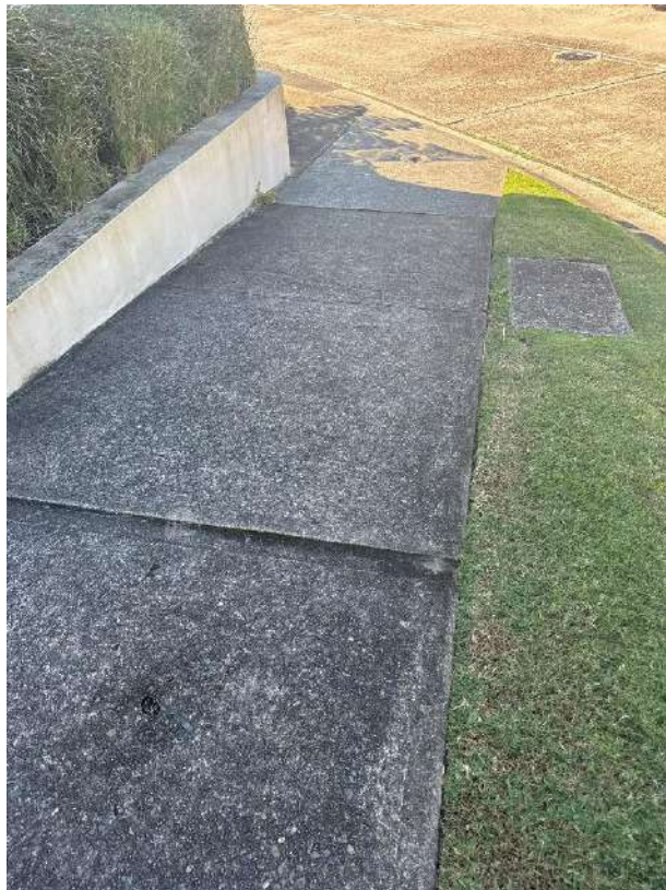
Cracks in the concrete foot path and elevated concrete pathway
