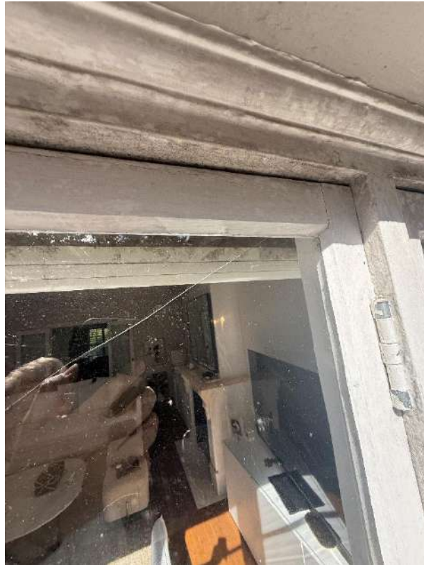
Cracked glass window pane
