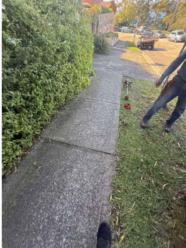
Elevated concrete pavement
