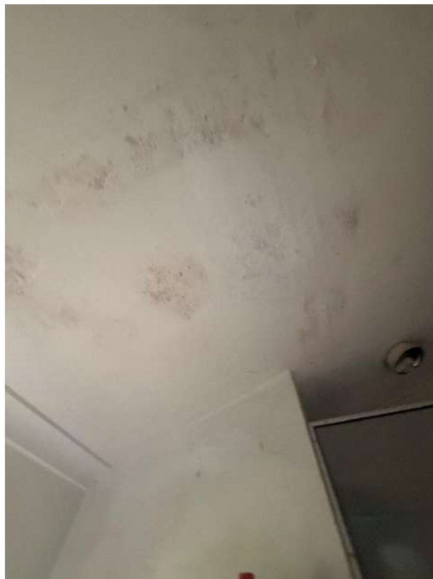
Moisture damage within the ceilings outside bathroom
