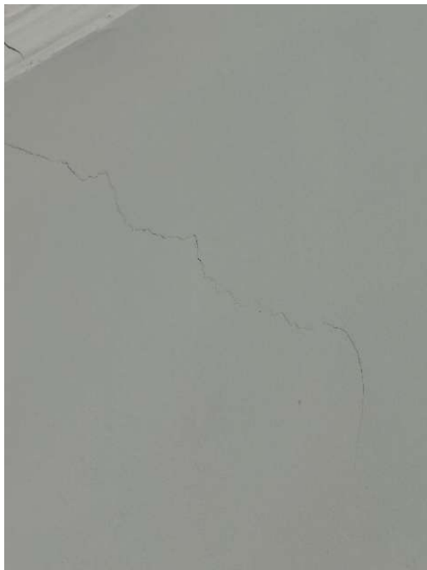
Splayed cracking within the living room walls
