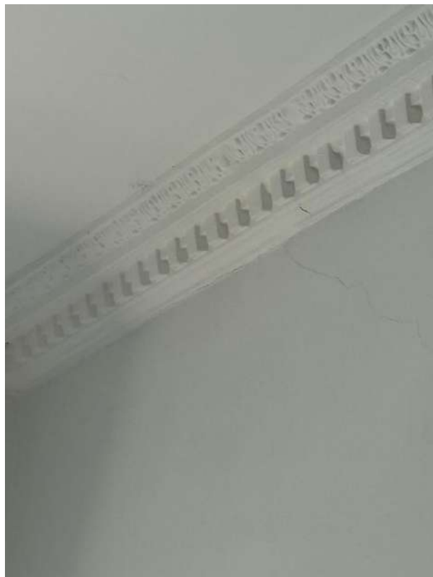
Splayed cracking within the living room walls
