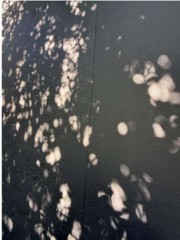
Vertical cracks seen within the external masonry walls running the whole length of the walls from floor to eave linings
