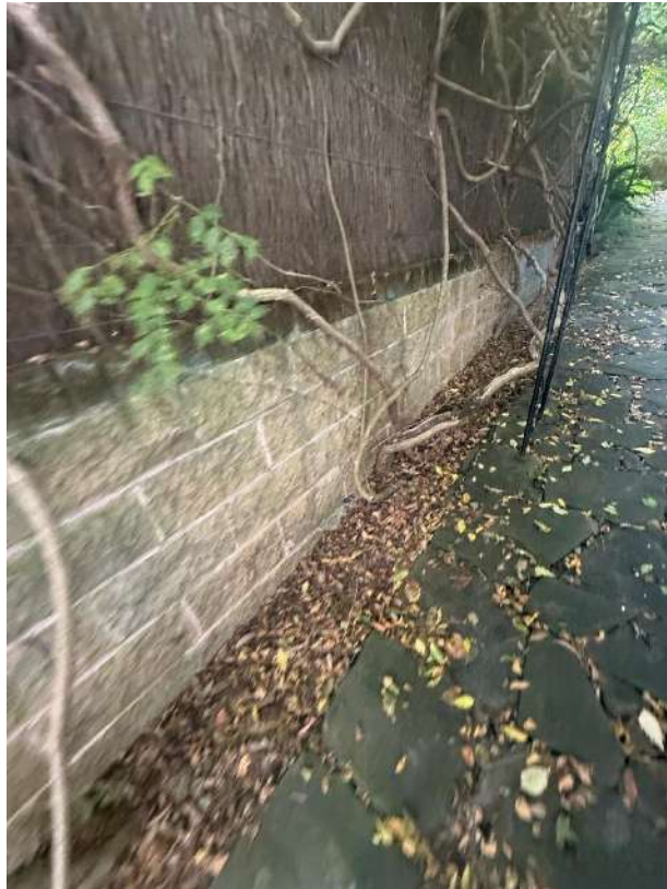
Cracks within the sandstones flagging floor finish
