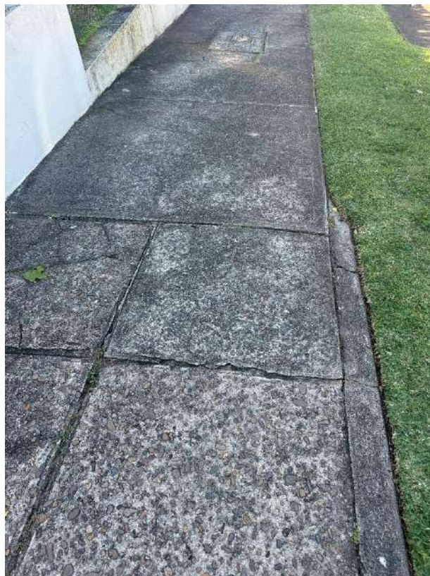
Cracks in the concrete foot path
