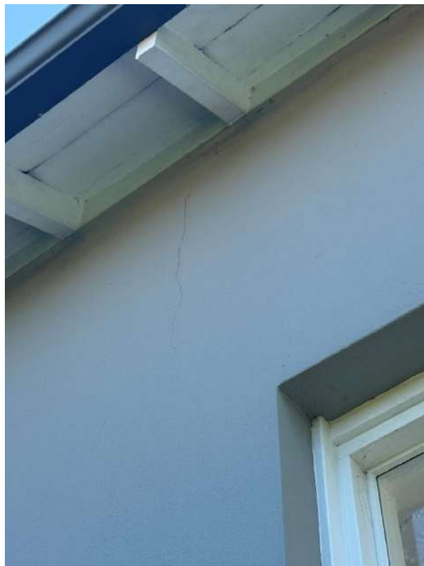
Top-left corner of the window has a vertical and horizontal crack within the external rendered wall
