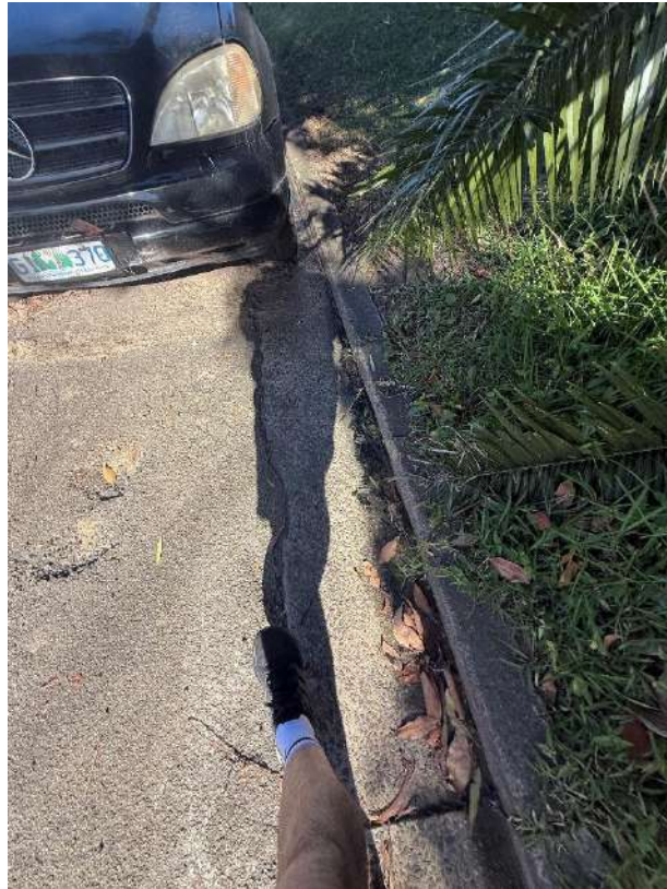
Minor cracks within the concrete curb and gutter
