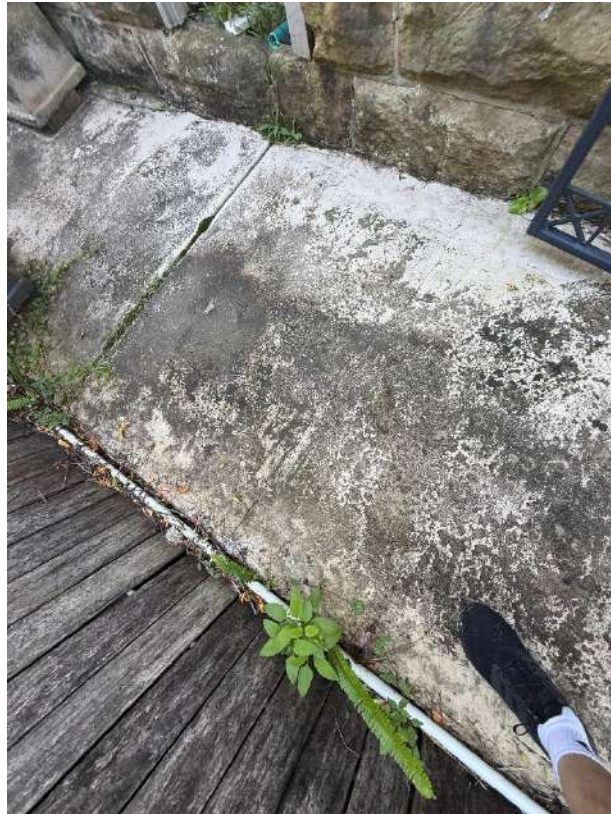
Cracks within the concrete left pathway
