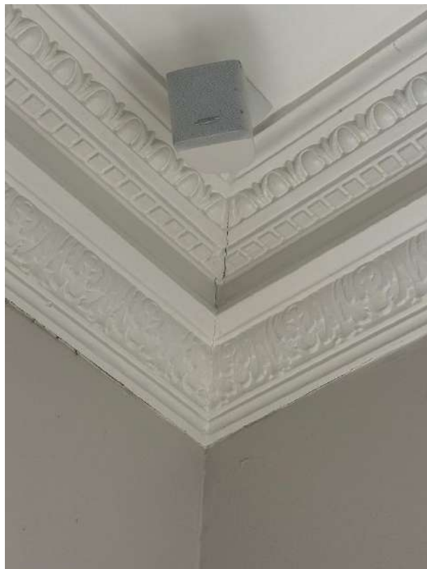
Minor hairline cracks seen within the cornices within the living room ceiling
