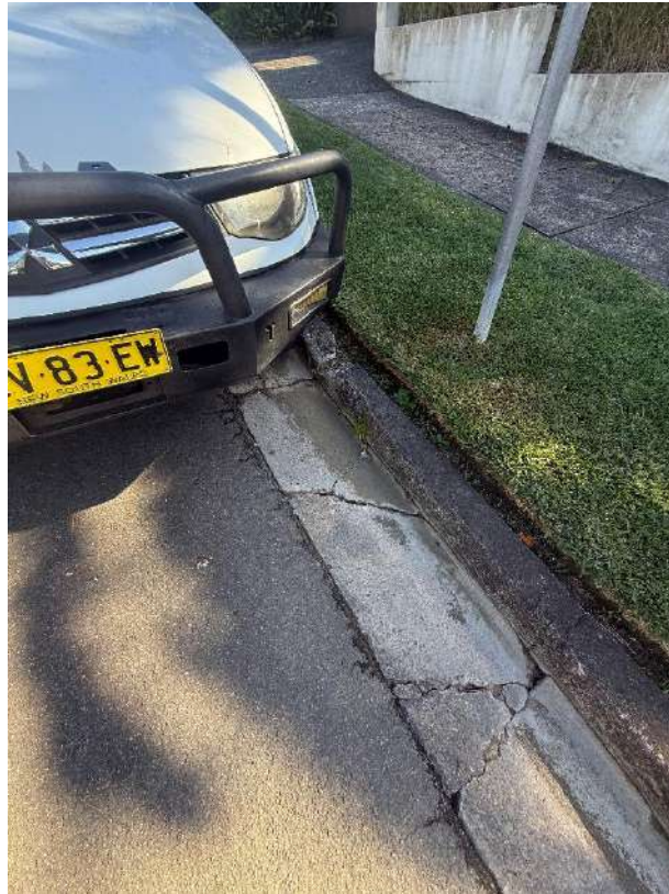
Considerable cracks in the concrete curb and gutter
