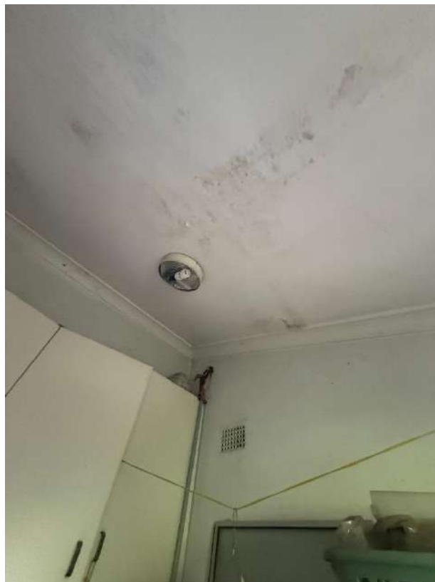
Moisture damage within the ceilings outside bathroom laundry
