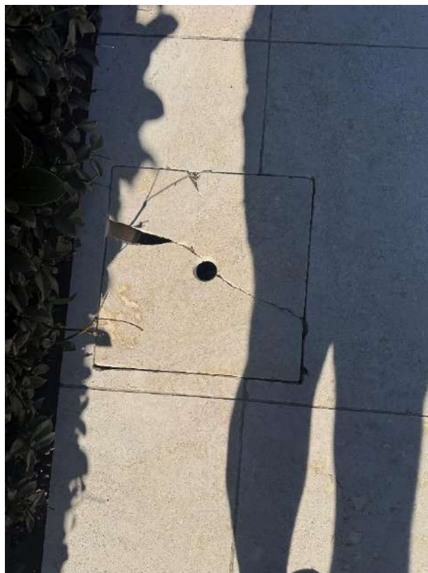
Cracks within the pool skimmer box cover
