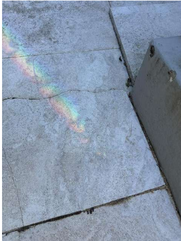
Elevated lifted drummy and cracked floor tiles and pathway
