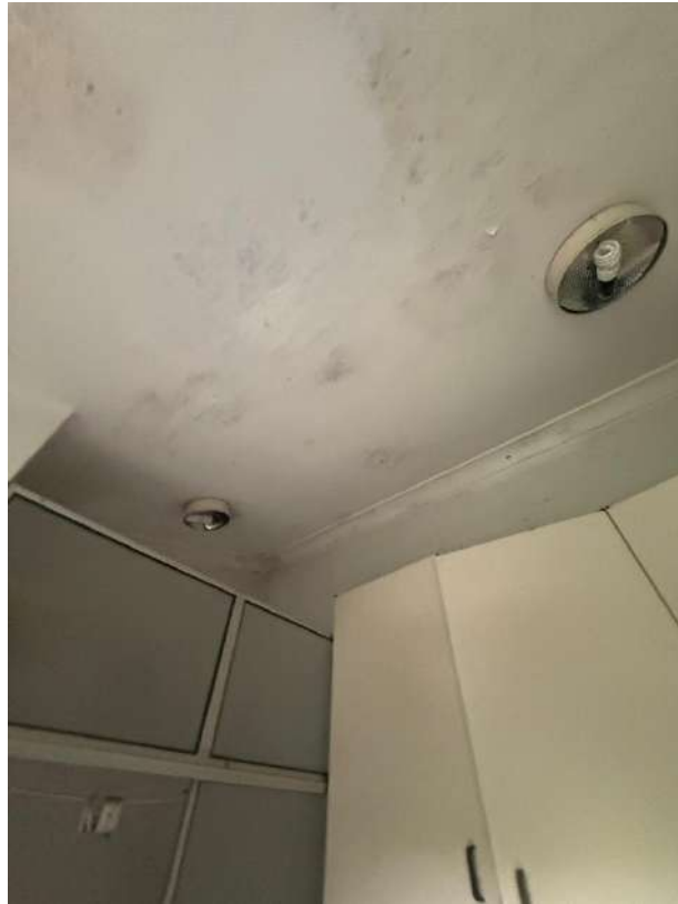
Moisture damage within the ceilings outside bathroom laundry
