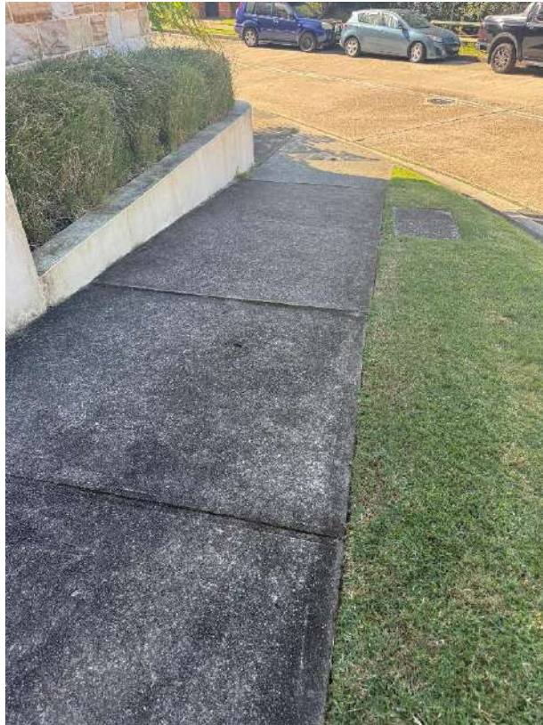
Cracks in the concrete foot path and elevated concrete pathway
