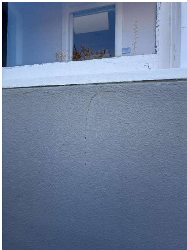
Horizontal and vertical cracks beneath the windows
