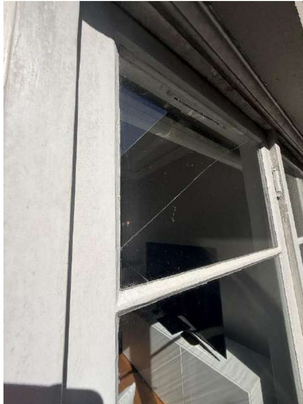
Cracked glass window pane
