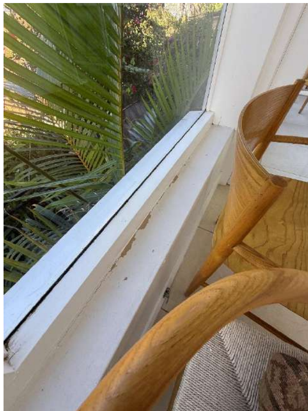
Moisture ingress within the sunroom and wall junction
