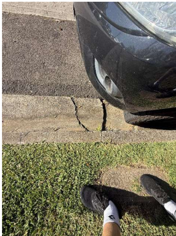
Cracks and damage within the curb and gutter
