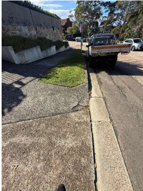
Cracks in the concrete driveway
