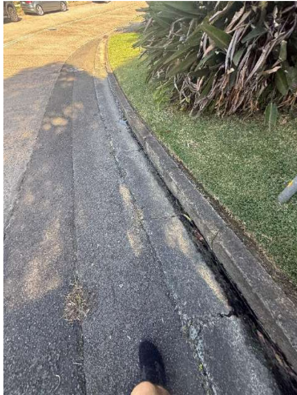
Wear and tear within the concrete curb and gutter
