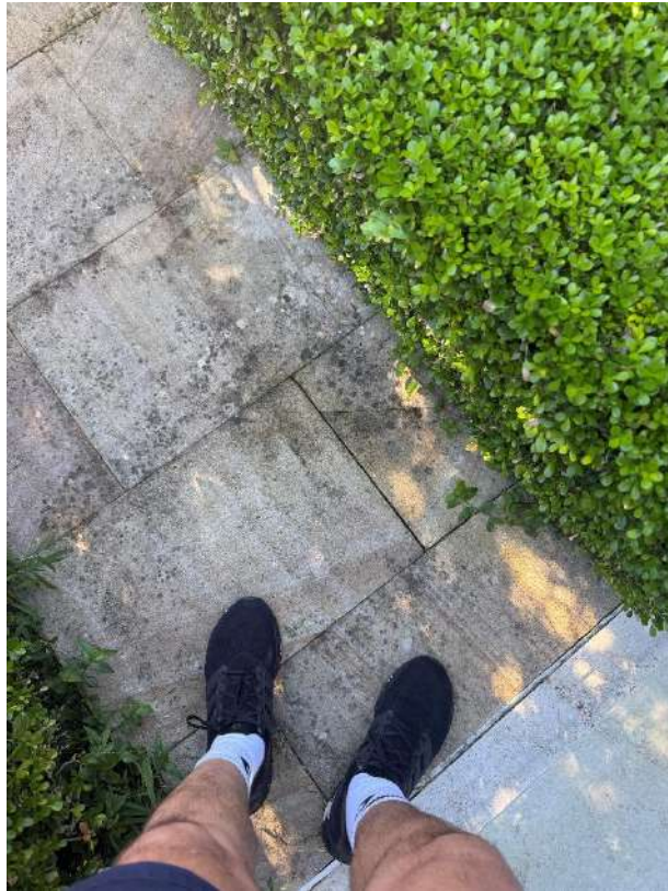
Pathway sandstone flagging cracks running through the sandstone pavers
