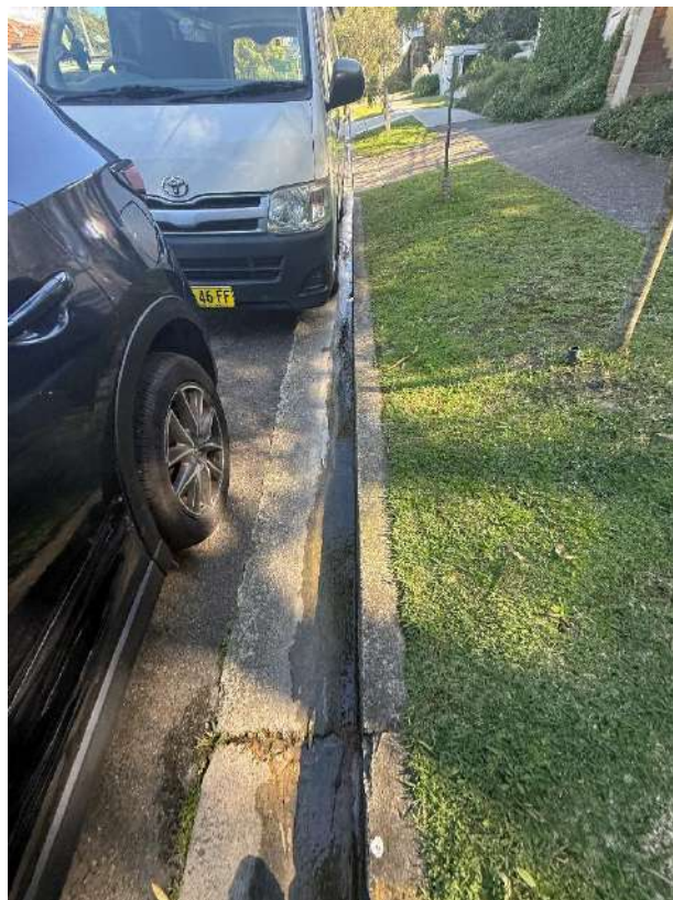
Considerable cracks within the concrete curb and gutter
