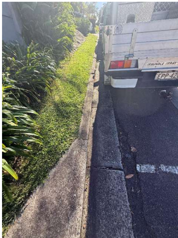
Cracks in curb and gutter
