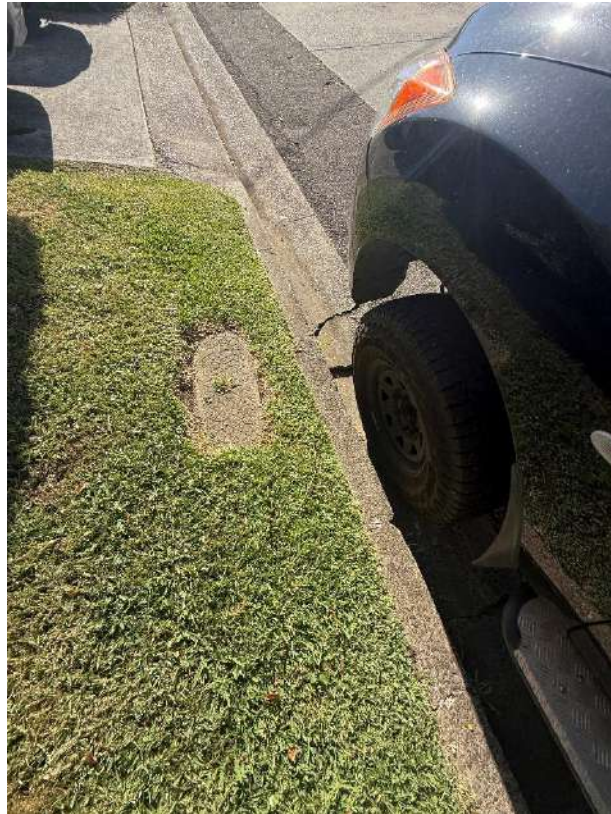
Cracks and damage within the curb and gutter
