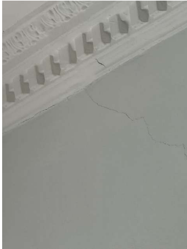
Splayed cracking within the living room walls
