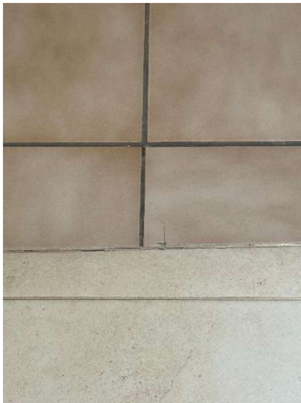
Crack in the floor tiles within the doorway of the laundry
