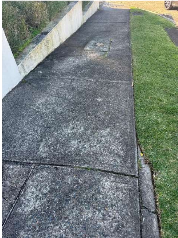
Cracks in the concrete foot path
