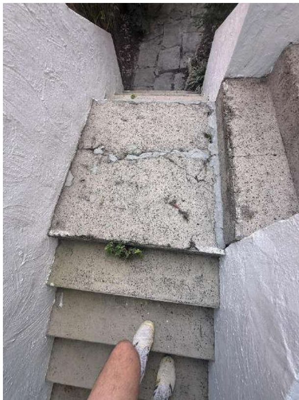
Considerable cracks within the entry stairs and landing leading to the front door
