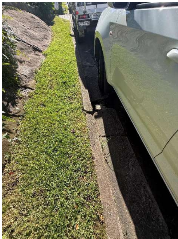
Cracks in curb and gutter
