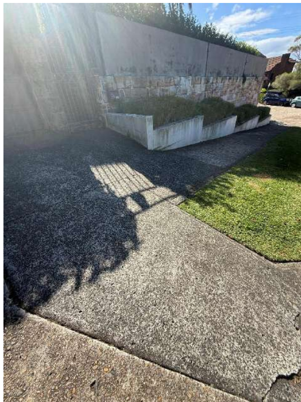
Cracks in the concrete driveway
