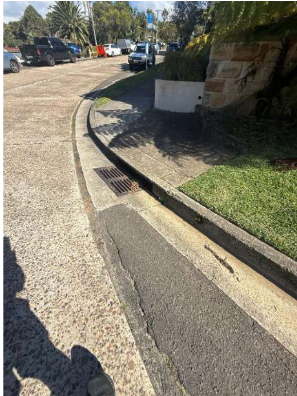
Bitumen cracked
