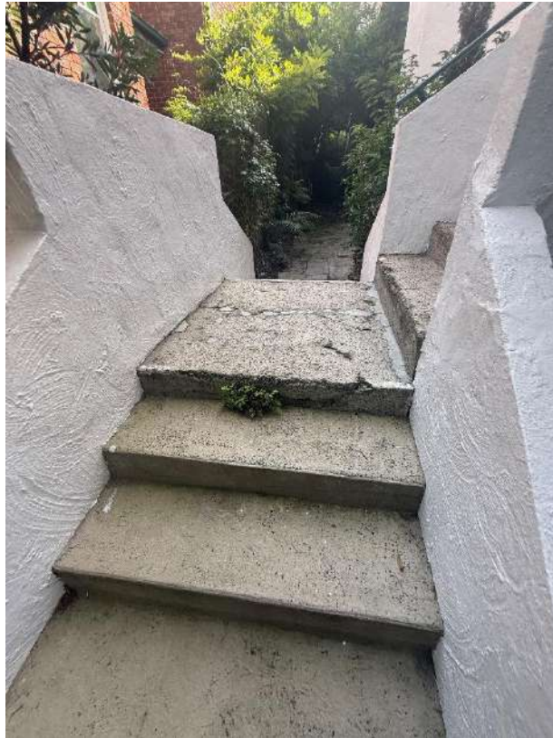
Considerable cracks within the entry stairs and landing leading to the front door
