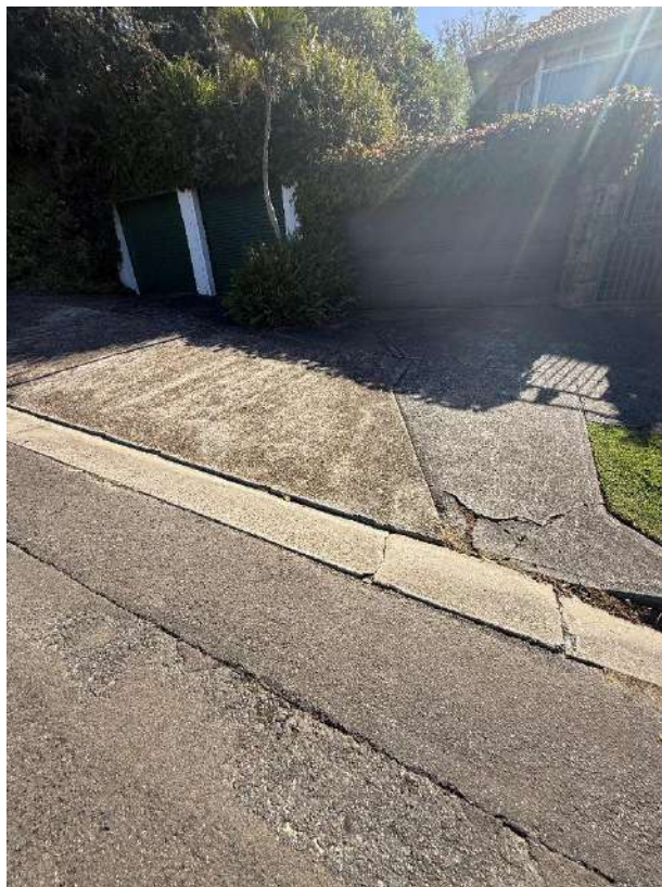
Road in poor condition and cracks within the concrete driveway and curb and gutter
