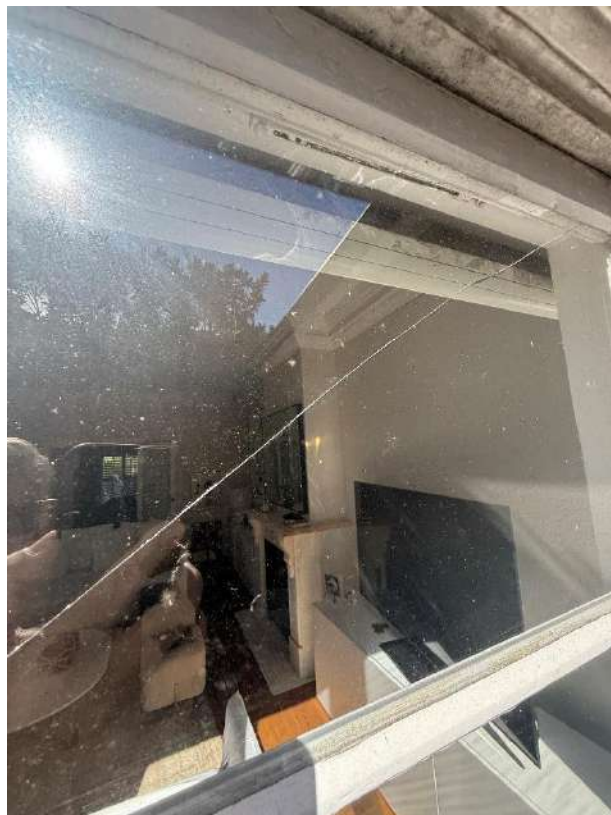
Cracked glass window pane
