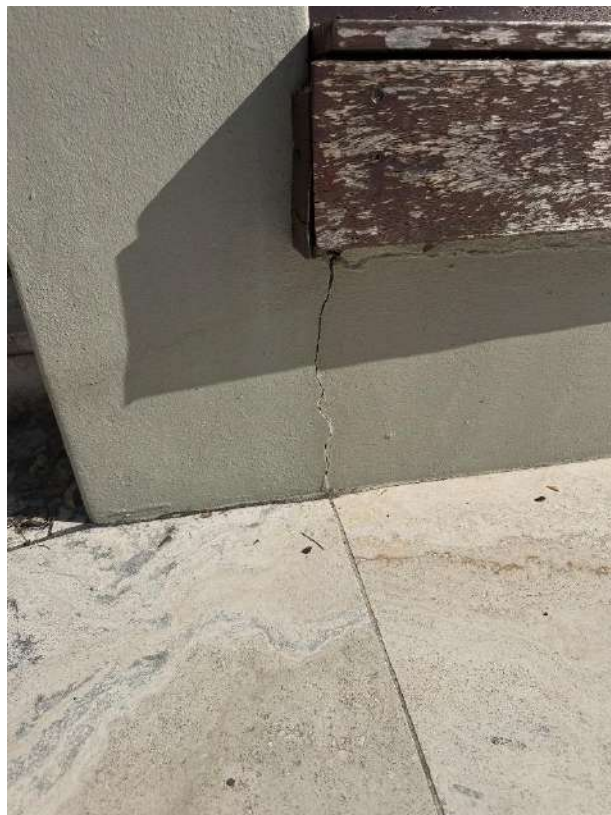
Retaining wall minor horizontal and vertical cracks within the render
