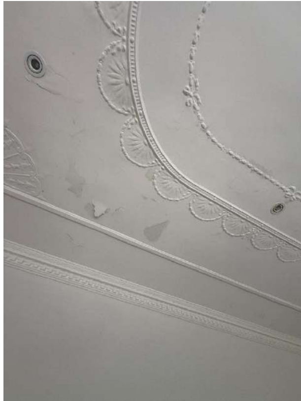
Peeling paint within the living room ceiling and cornices
