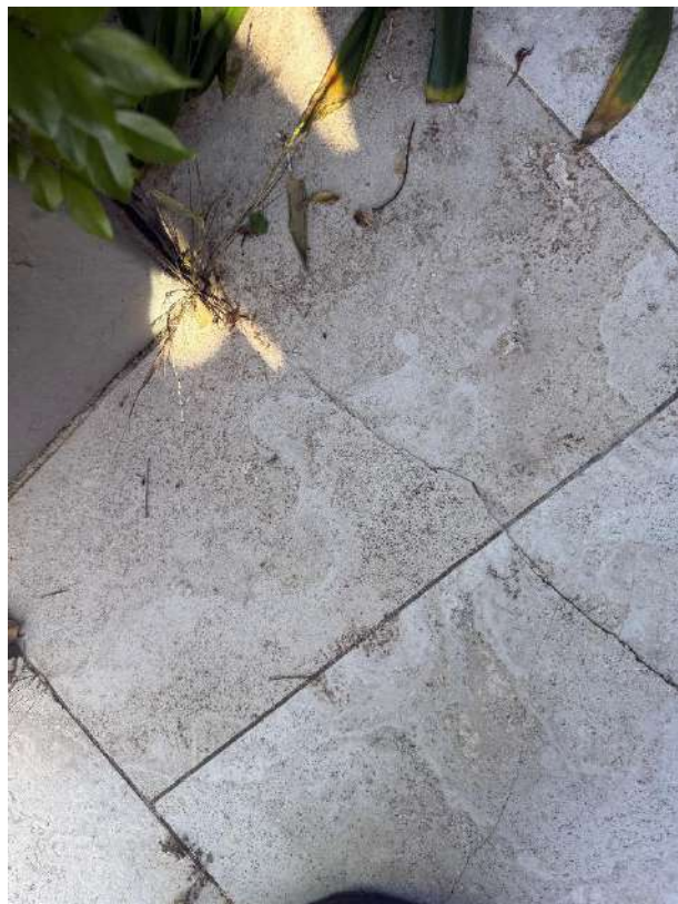
Elevated lifted drummy and cracked floor tiles and pathway
