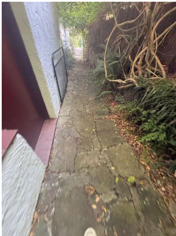
Cracks within the sandstone mortar joints
