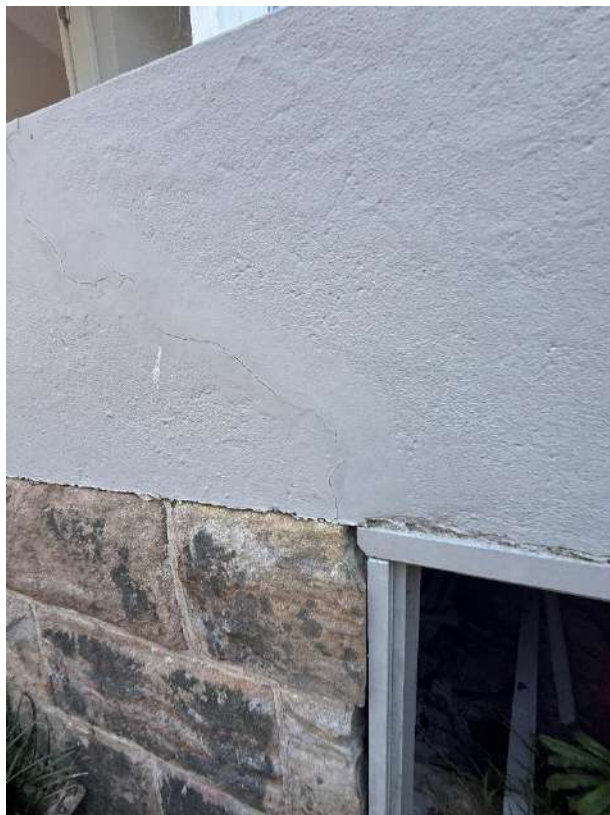
Left elevation of the wall has splayed cracking in the masonry walls
