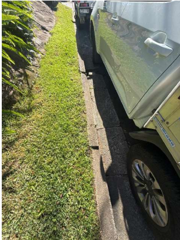
Cracks in curb and gutter
