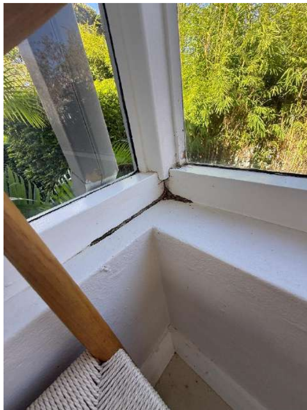
Water ingress within the sunroom window and masonry wall junction
