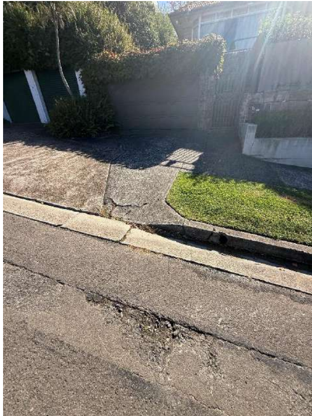
Road in poor condition and cracks within the concrete driveway and curb and gutter
