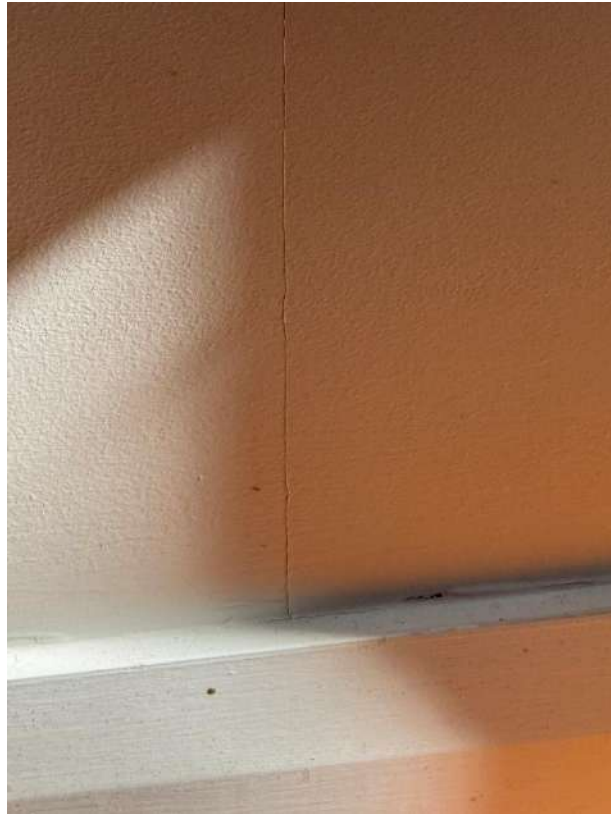
Horizontal cracking within the back office beneath the window frame
