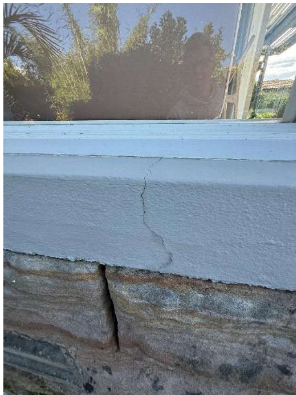
Crack within the external rendered wall below the window
